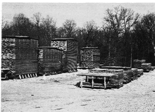
Figure 15. (Left) The sawmill that was located at the Kaskaskia Experimental Forest from 1950 to 1971 (this photo was taken during the Southern Illinois University Forestry Camp held at the Forest May 15-19, 1961, and shows a student operating the headsaw) and (Right) the KEF air-seasoning yard in 1961 showing roofed and unroofed piles of lumber.
