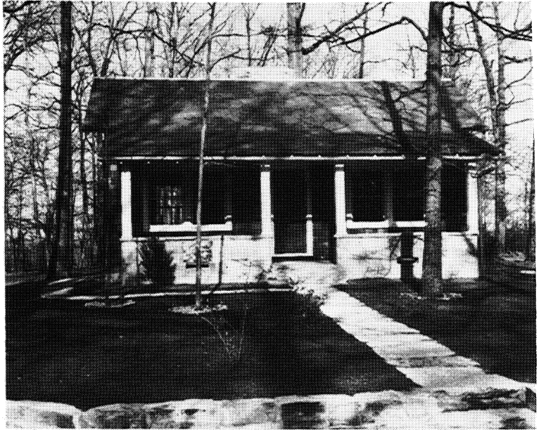
Figure 5. The 5-room dwelling constructed at the Kaskaskia Experimental Forest for the Supervisor.
