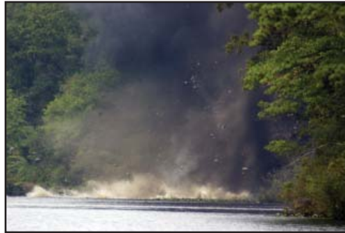
(Right) Sgt. Erich Wagner, second class diver, pulls detonation from one of two points. Divers must tape C4 plastic explosives to obstacles underwater and, in murky water like Fort A.P. Hill, do so with limited visibility. (Above) Army divers successfully eliminate a water obstacle.
