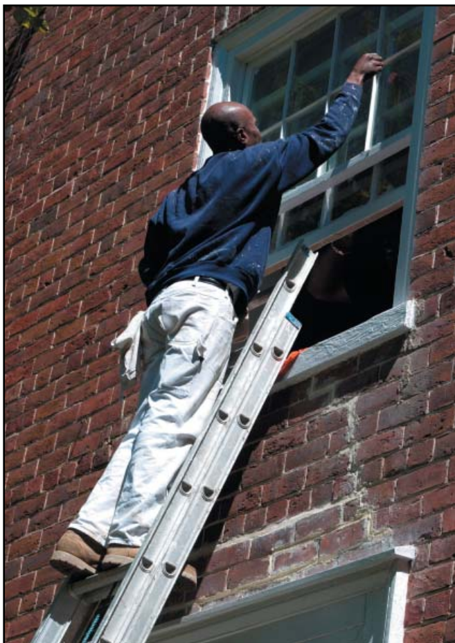
Liberty Church is currently being renovated. Renovations include brick replacement, repainting window panes and replacing the roof. (Photo by Mary A. Bodine)
