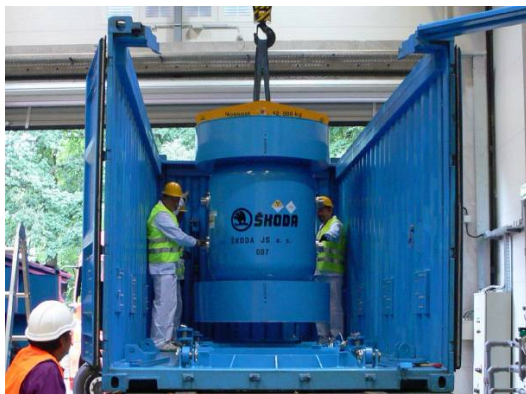
Fig. 5. SKODA VPVR/M cask is installed into ISO-container
