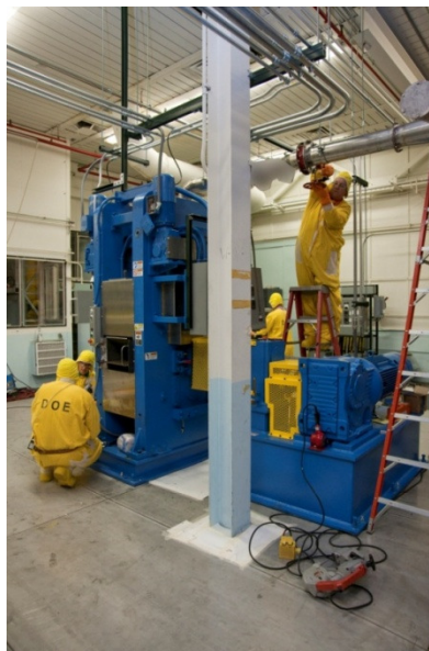
Figure 9: Installation of New Rolling Mill
