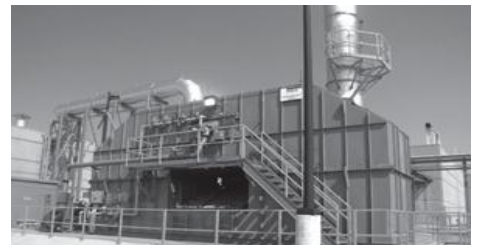
In support of the “Clean Texas Program,” the WCF installed a high efficiency Regenerative Thermal Oxidizer (RTO). The RTO is used for the treatment of exhaust air and is instrumental in the reduction of air pollution at the WCF.
