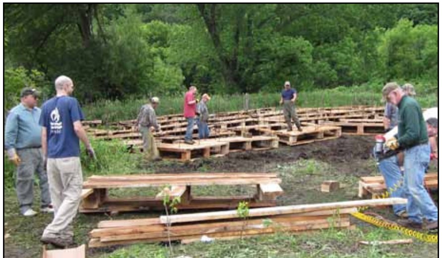
A work party building lunkers structures that will be installed into the streambank to create habitat for fish in the newly restored stretch of Bear Creek.
