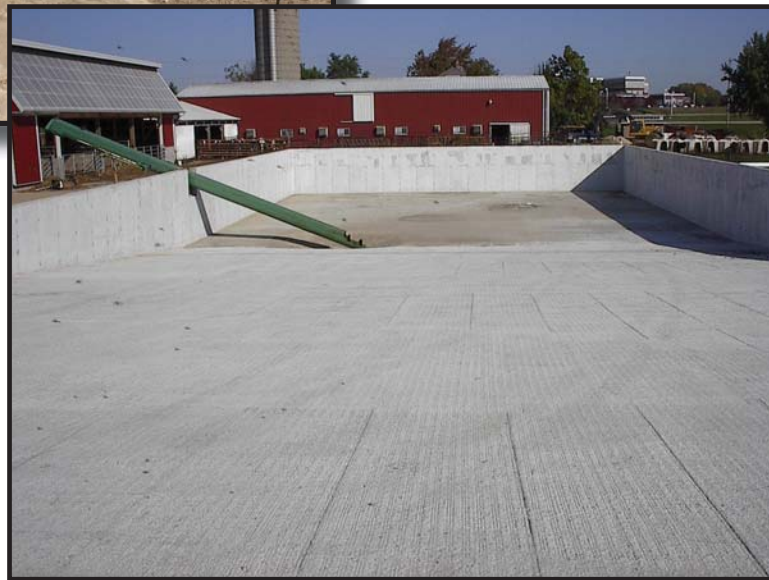
After photo: A waste storage facility allows the farmer to spread manure safely during optimum weather, thereby reducing risk of runoff, and at the best time and place for the crop to utilize the nutrients in the manure.
