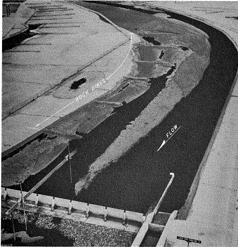
Fig. 2. Channel development upstream of a lock and dam. Water Surface lowered to 14 ft below normal pool
