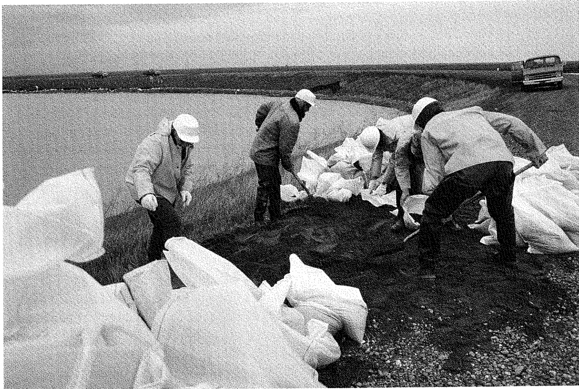
Sand bagging on major river levee. Photo courtesy California DWR.
