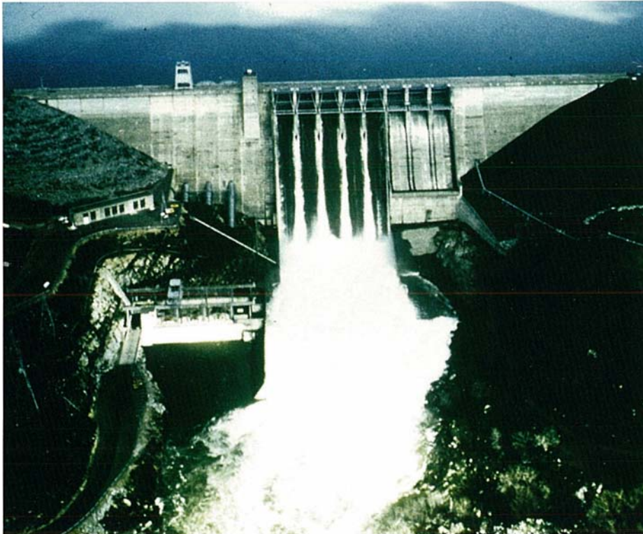
Folsom Dam, American River, California
