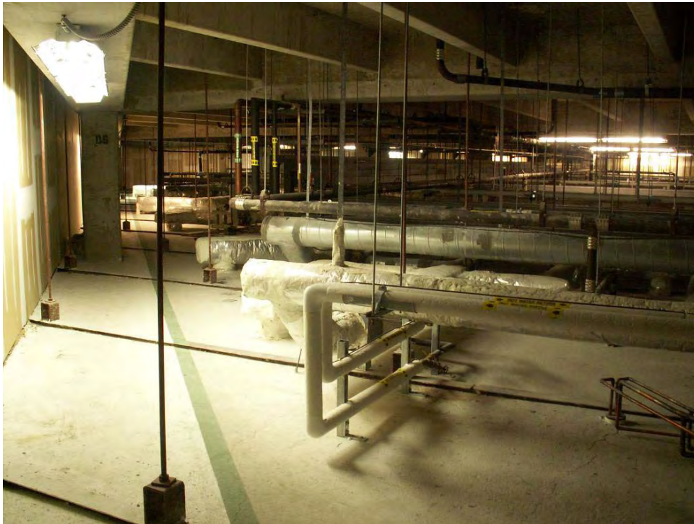
Photo C-4 Interstitial Service Zone
