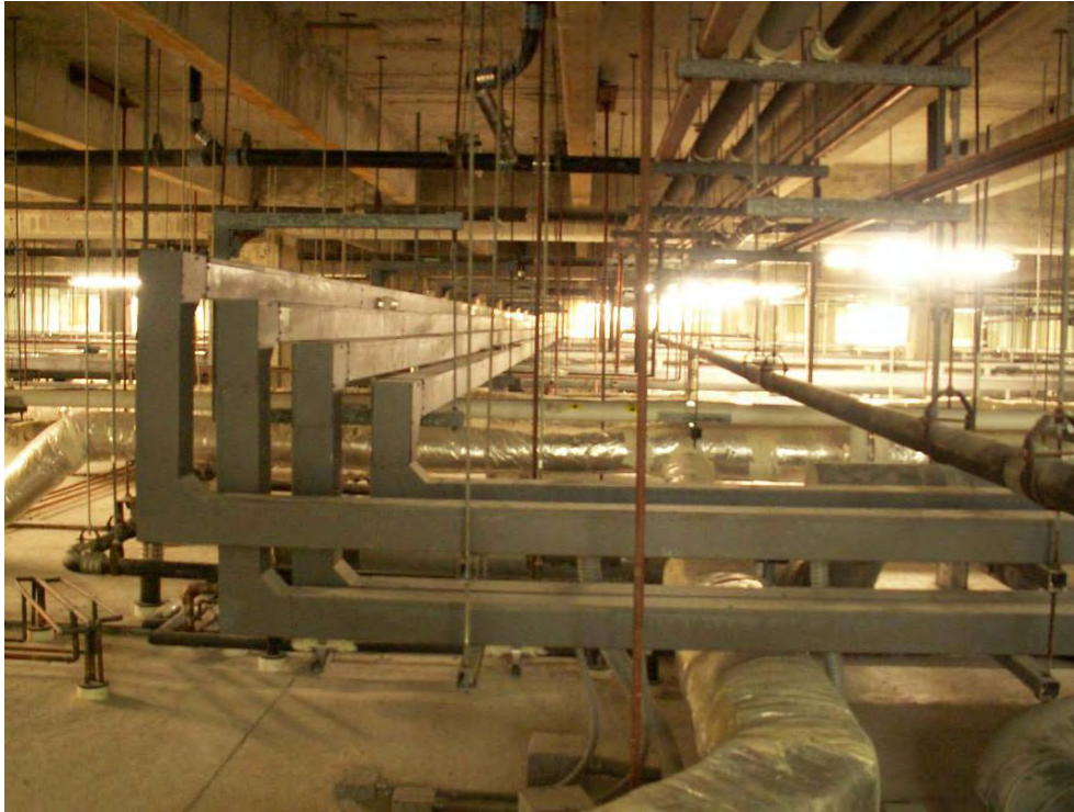
Photo C-5 Interstitial Service Zone Showing typical distribution
