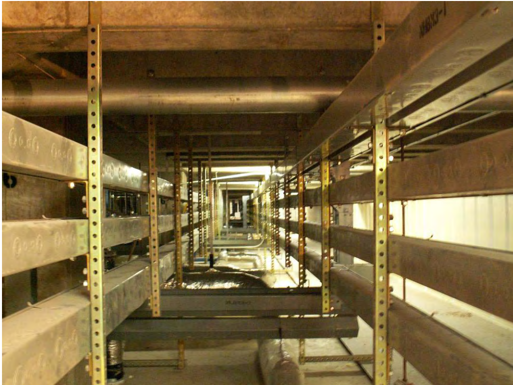
Photo B-3 Showing wireways in S-3 and S-4 subzones
