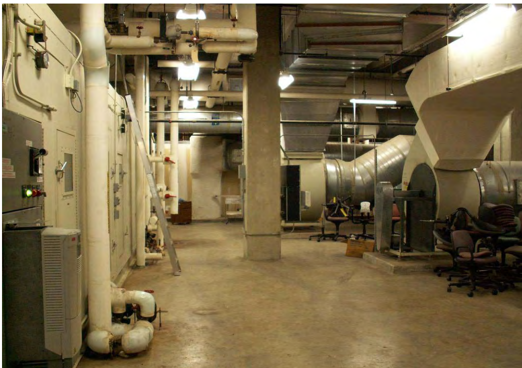
Photo B-4 Typical Service Bay
