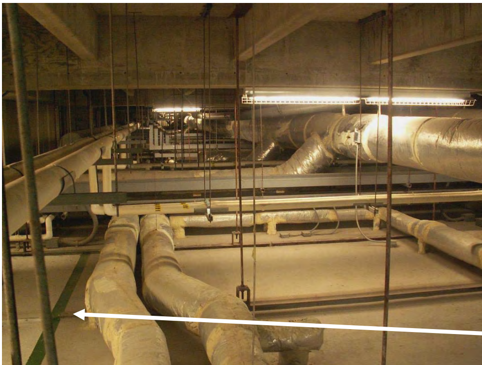
Photo C-8 Interstitial Service Zone
