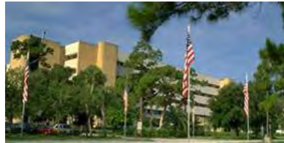
VA Medical Center Bay Pines, FL, 1983
