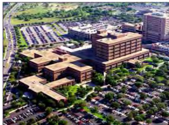
VA Medical Center San Antonio, TX, 1973 (not VAHBS, but used interstitial space)
