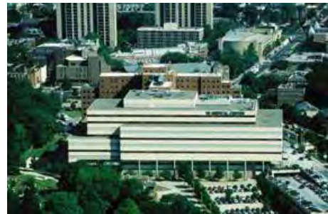
VA Medical Center Philadelphia, PA, 1994 (not VAHBS, used interstitial space)
