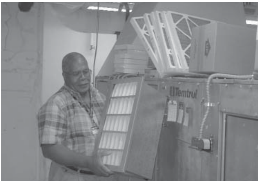
Building equipment maintenance
