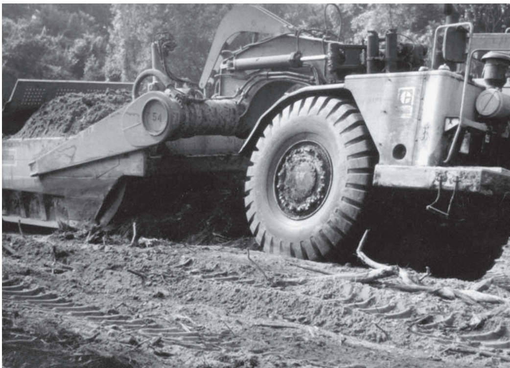
Figure 9.4. Scrapers are useful for short-distance transport of topsoil.
