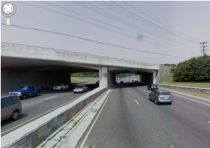
MD 193 Bridge (Northbound)
