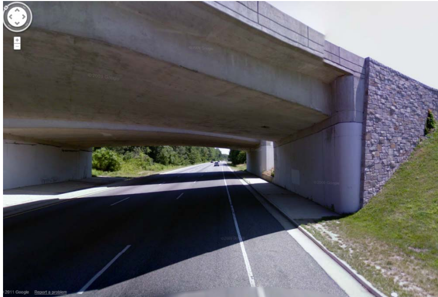
MD 198 Bridge (Northbound)
