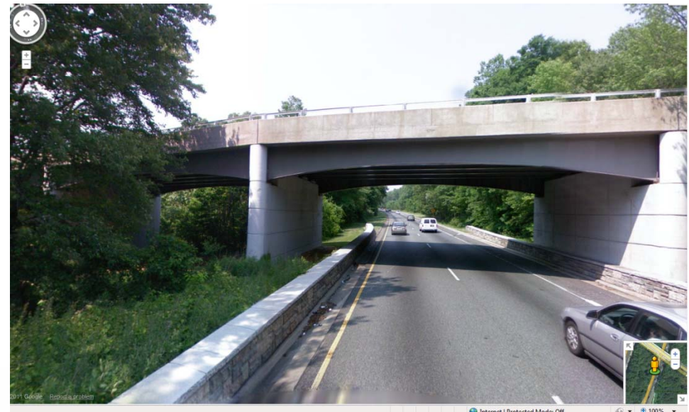
Explorer Rd Bridge (Northbound)
