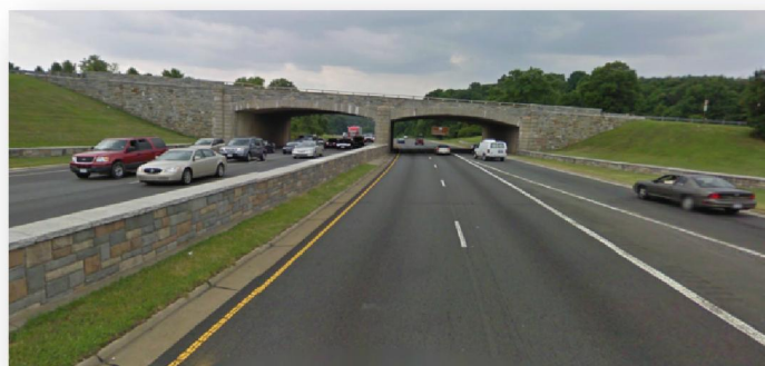
MD 450 Bridge would require reconstruction
