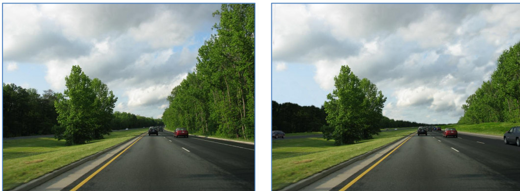
Before After Figure 3.7. AASHTO/SHA Outside Widening Option
