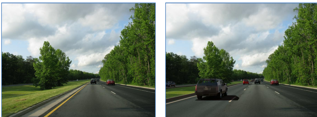
Before After Figure 3.8. NPS Inside Widening Option
