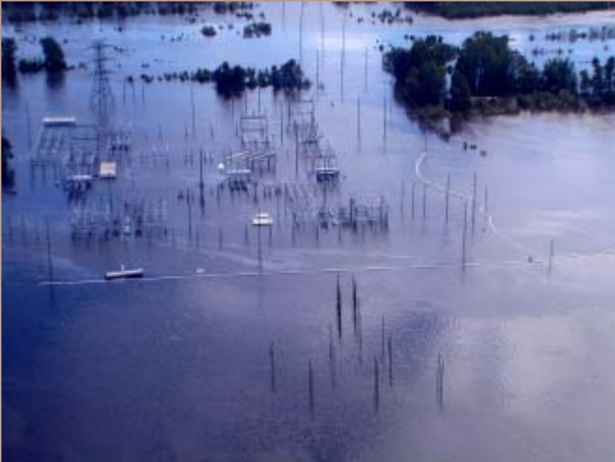
Flooded Power Plant in North Carolina during Hurricane Floyd, 1999
