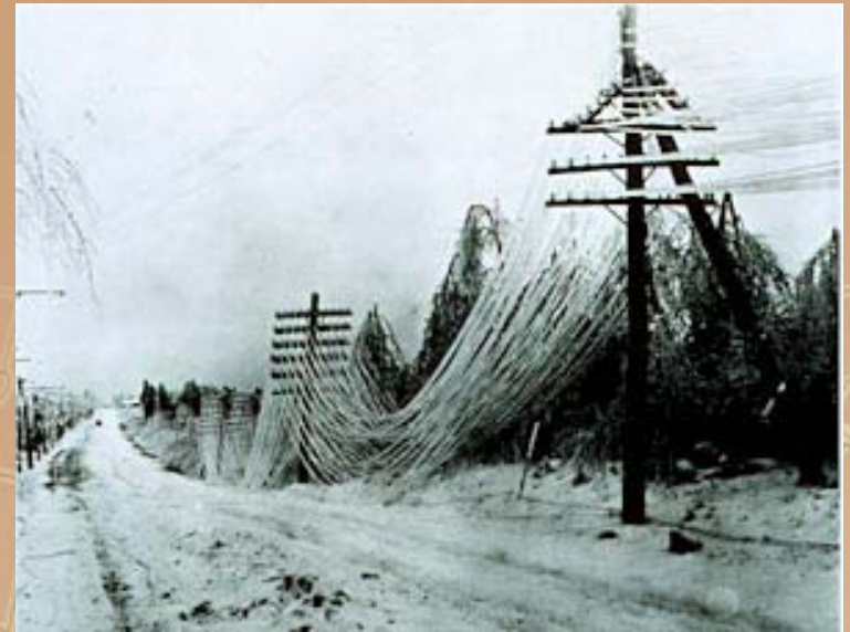
Ice Storm Causing Downed Power Lines
