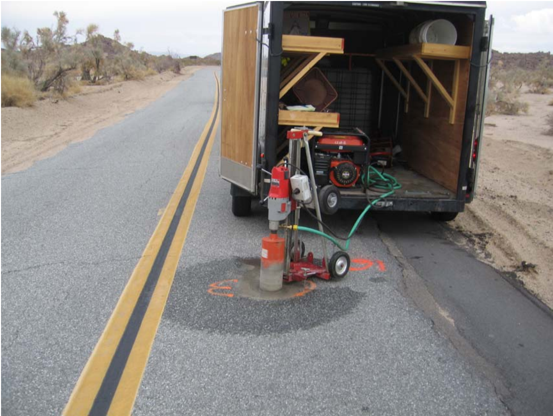
Edge repair at core 16
