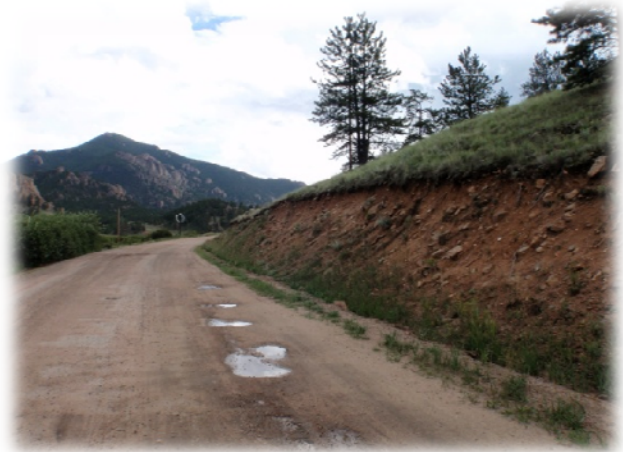
FIGURE 3:- Station 1672 Typical Cutslope Brow
