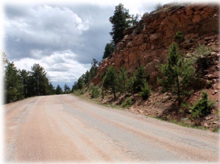
FIGURE 1:- Station 1689+50 Rock Cut
