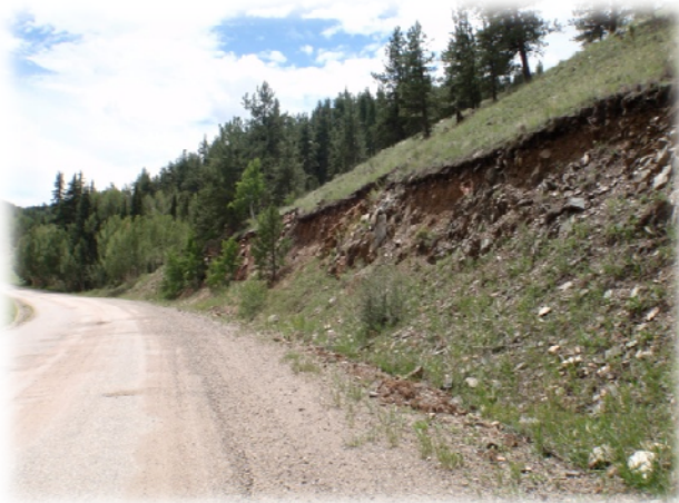
FIGURE 2 Station 1592 Typical Cutslope Brow
