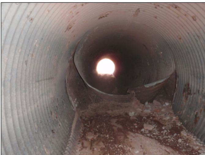
Sta 324+54 72" CMP failed joint (view upstream) before temporary repair (left) and after repair (right)
