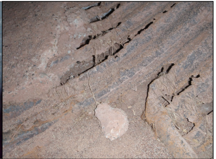
Sta 324+54 72" CMP corrosion and perforation and invert deterioration
