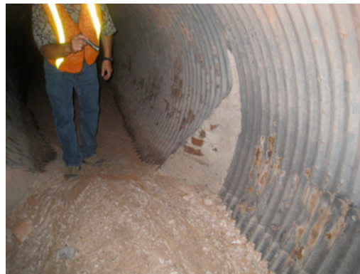
72” Culvert Repaired Joint
