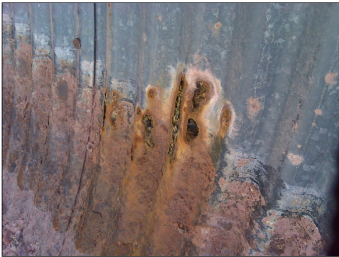
Sta 324+54 72" CMP corrosion and perforation and invert deterioration
