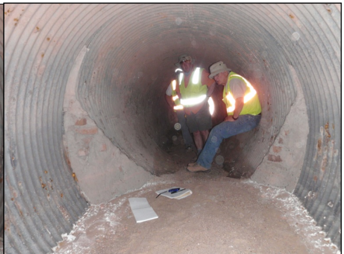
Sta 324+54 72" CMP failed joint (view upstream) before temporary repair (left) and after repair (right)
