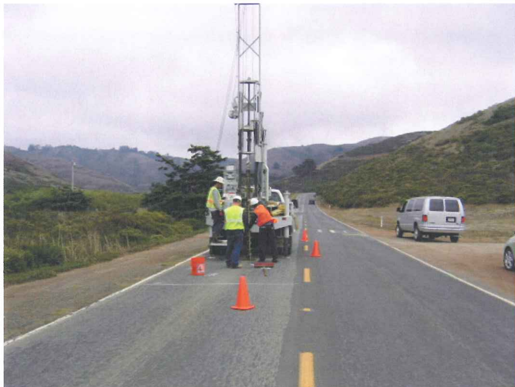
MP 1.32 Bunker Road, B-16 looking east
