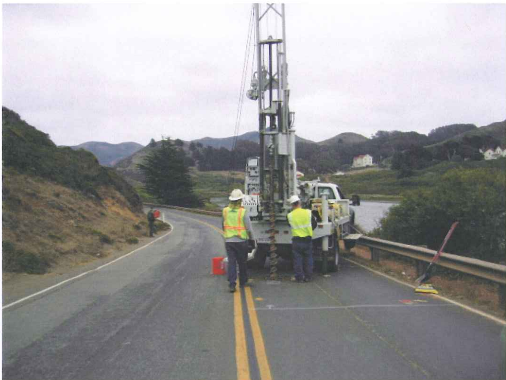
MP 0.02 Bunker Road, B-42 looking east
