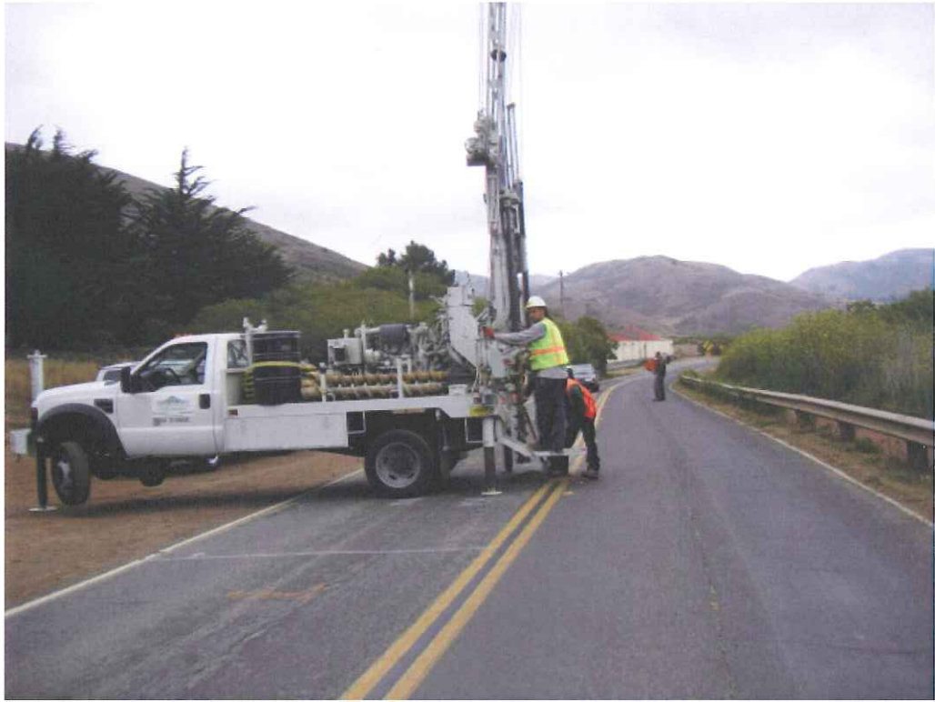
MP 0.11 Bunker Road, B-12 looking east
