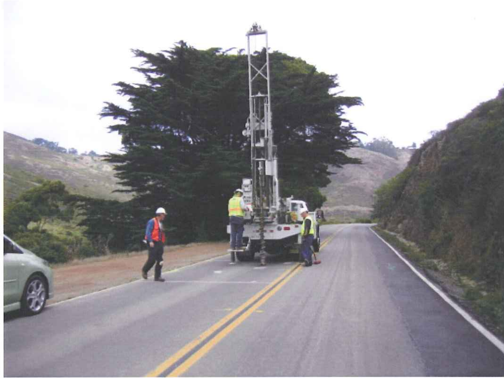
MP 2.18 Bunker Road, B-28 looking east, note utility cut right
