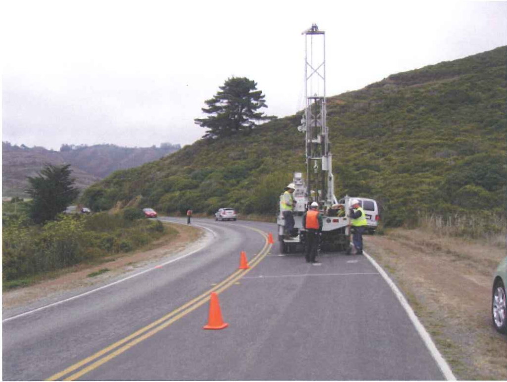
MP1.61 Bunker Road, B-17 looking east
