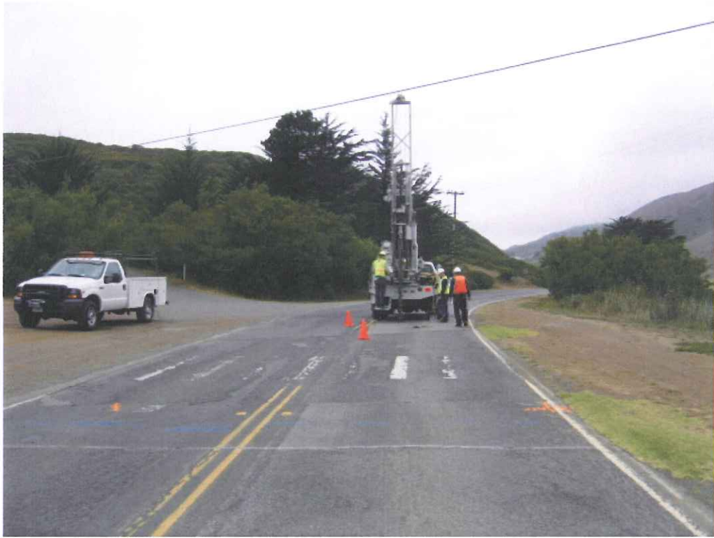
MP 0.70 Bunker Road, B-14 near the equestrian area, looking west
