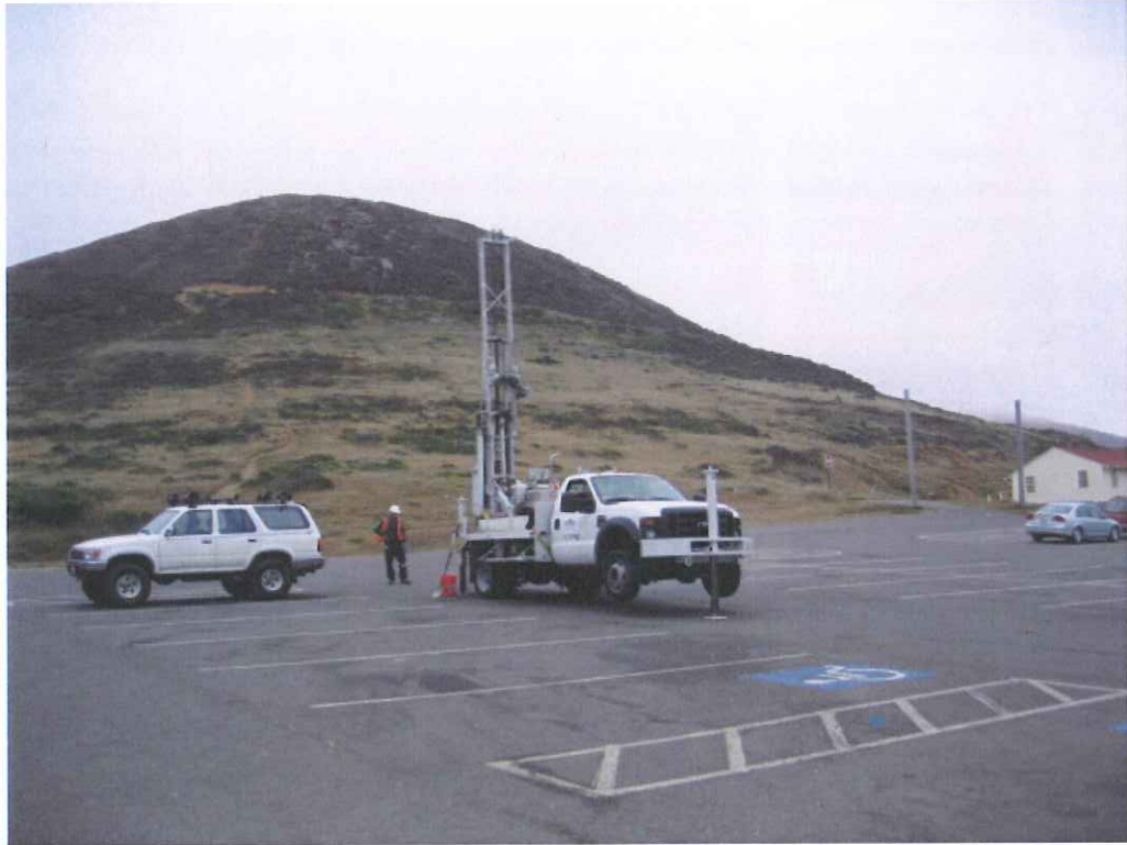
MP 0.08 Mitchell Road, informally called Surfer Parking, looking north
