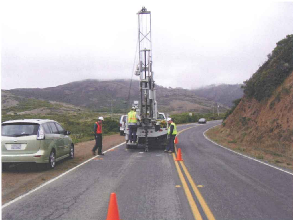
MP 1.72 Bunker Road, B-18 looking east
