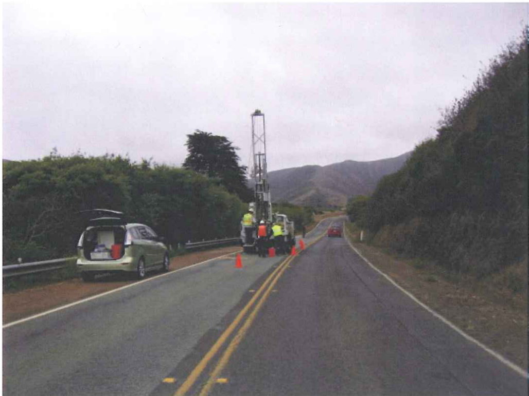
MP 0.32 Bunker Road, B-9 looking east
