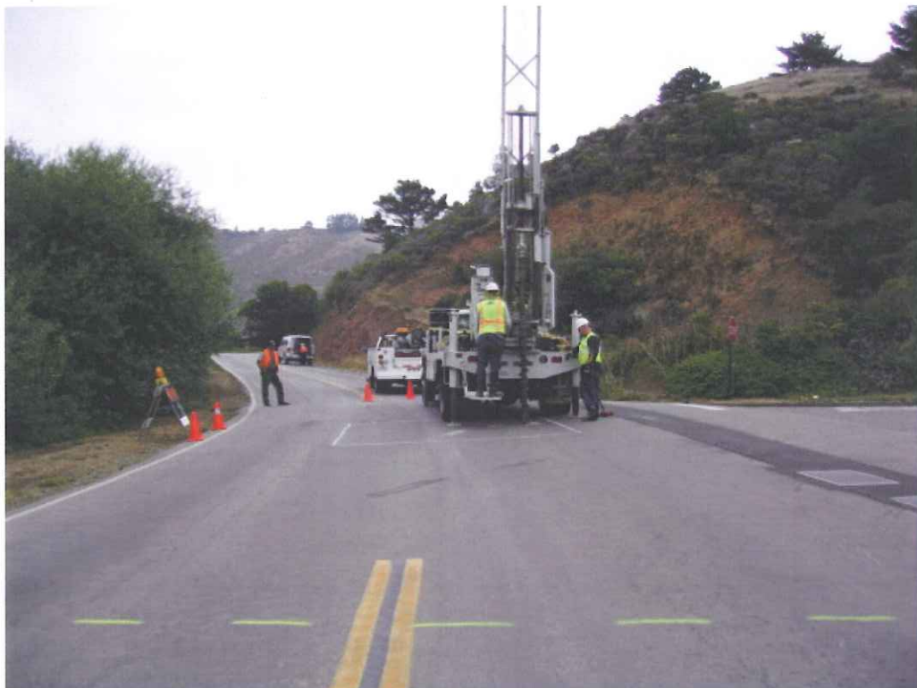
MP 2.09 Bunker Road, B-57 looking east, note utility cut right
