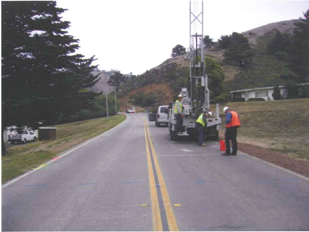
MP 2.02 Bunker Road B-27 by Intersection with McCullough Road, looking east
