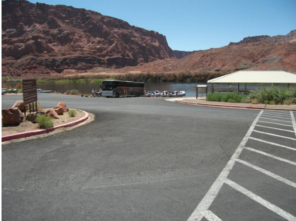
Photo 10 - Launch area with bus recently slurry sealed, good pavement condition
