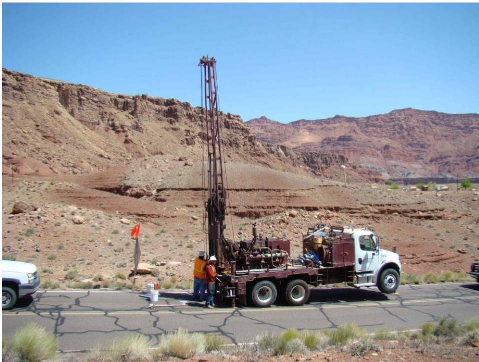
Photo 6 - Drilling P-16 with extensive block cracking
