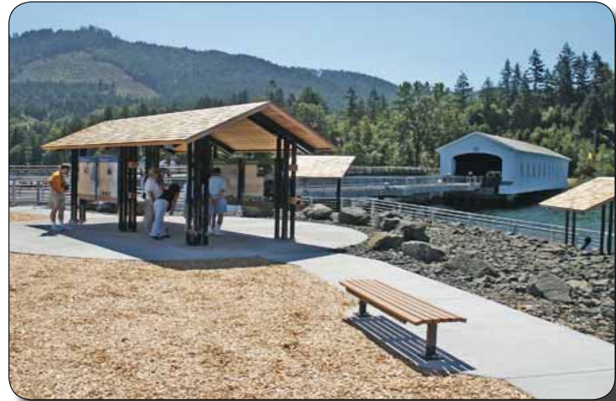
Lowell Covered Bridge, OR
