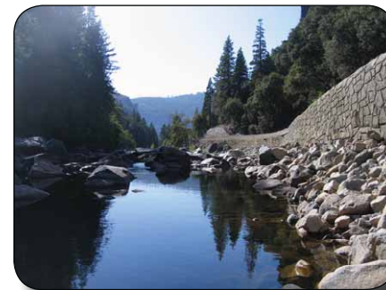
left to right: Highway improvement, Beartooth Highway, National Scenic Byway, Yellowstone National Park, MT; Bridge reconstruction, Natchez Trace Parkway, National Scenic Byway, TN; Aesthetic retaining wall, Merced River, Yosemite National Park, CA
