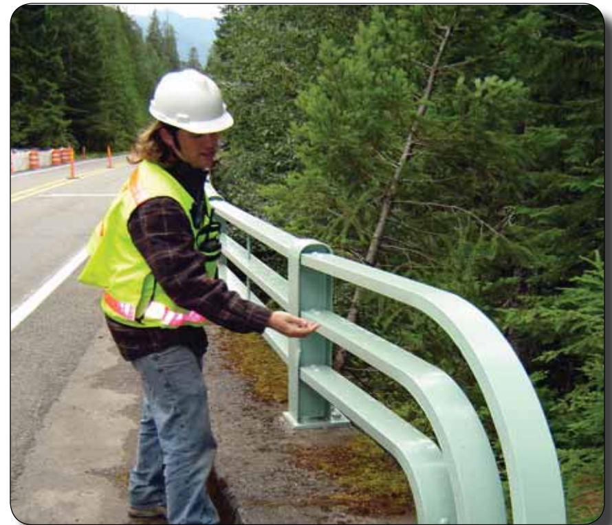
SCEP Employee, Bridge Inspection, Mt Ranier, WA
