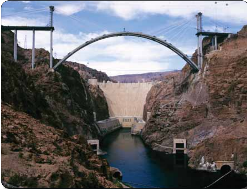
Hoover Dam Bypass, AZ & NV
