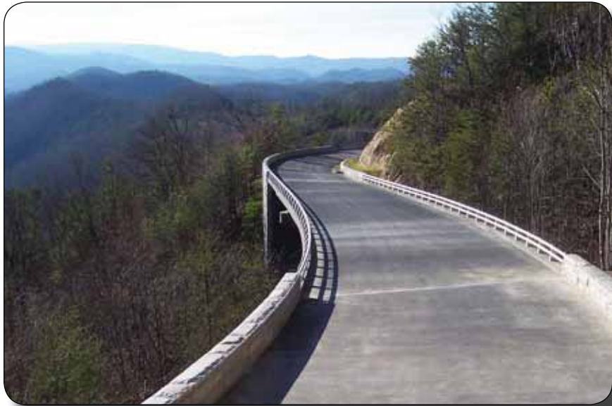
Foothills Parkway Bridge 8, TN
