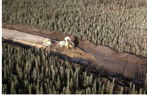
FIGURE 2.1-7 Trench Backfilling Operations (Source: TAPS 2007)
