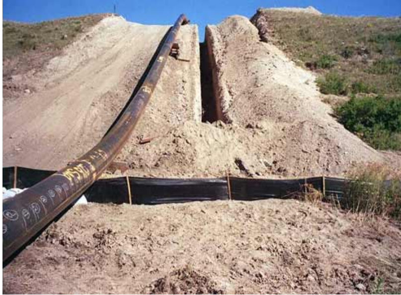
FIGURE 1.2-1 Typical Installation of a Large Transmission Natural Gas Pipe (Source: Argonne Staff)
