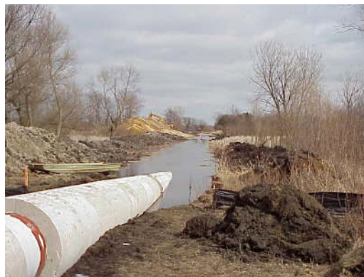
FIGURE 2.2-6 Pipeline for Wetland Installation Encased in Concrete to Counteract Positive Buoyancy (Source: Photo courtesy of U.S. Pipeline, Inc. Reproduced with permission.)
