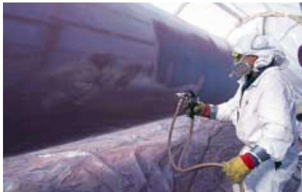
FIGURE 4.1-5 Crew Coating a Pipeline Field Joint (Source: TAPS 2001)
