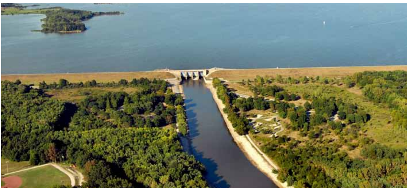
Aerial of the Carlyle Lake Dam. Photo by Allan Dooley.
