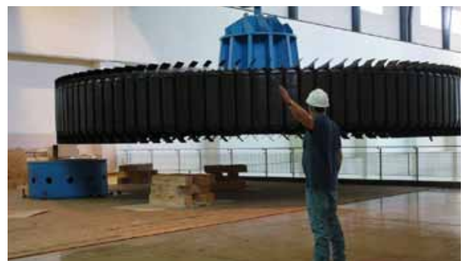
Guiding a 270-ton rotor assembly onto a pedestal at the Barkley Dam Hydropower Plant. U.S. Army Corps of Engineers photo by Lee Roberts.
