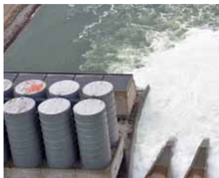
Garrison Dam releasing water into the Missouri River. North Dakota National Guard photo by Bill Prokopyk.
