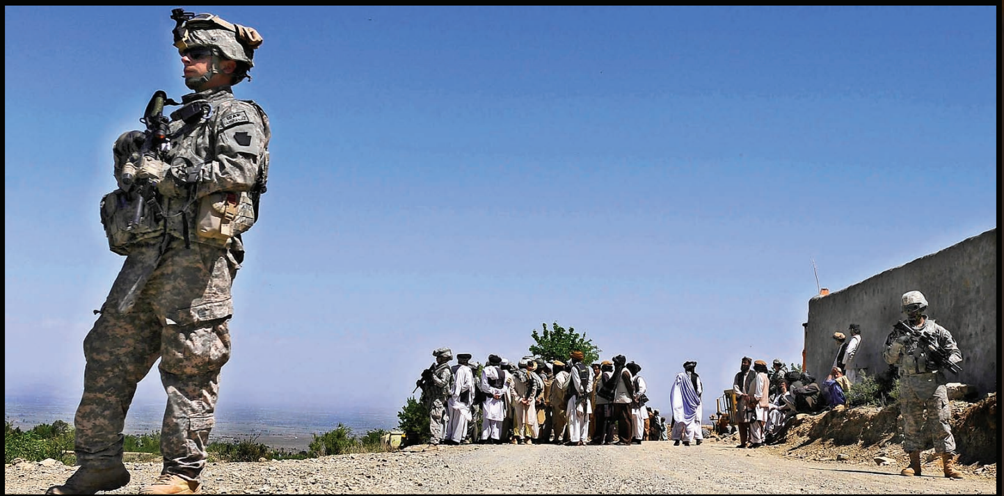
▲ Cpl. Shane Rager, left, provides security during a quality assurance check of the new road that extends from the Tani district center to Narizah village in Khost province, Afghanistan. Rager is an infantryman assigned to the Khost Provincial Reconstruction Team. The new road will provide a safer and more efficient route through the countryside. Photo by U.S. Air Force Senior Airman Julianne M. Showalter
