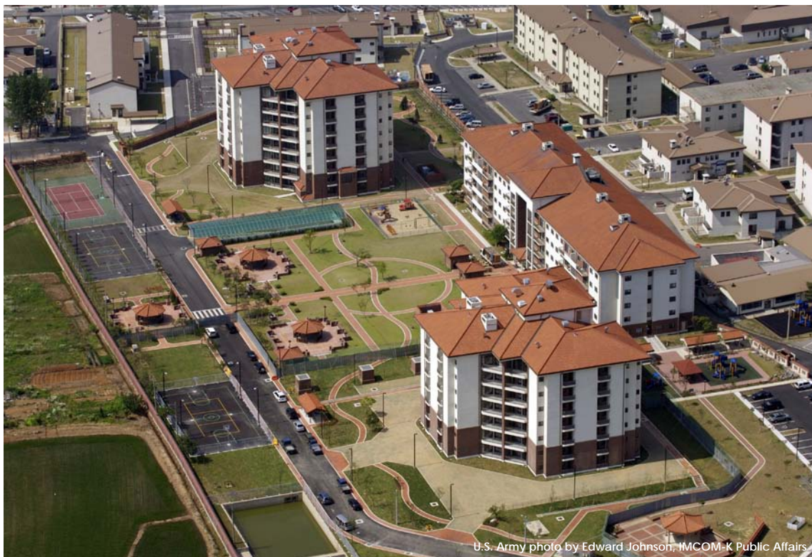
USAG Humphreys is leading the way in providing modern housing units for Soldiers and families stationed in Korea. The $8.3 billion expansion and construction effort will increase its capacity from 9,000 Soldiers, civilians and family members to more than 45,000.
