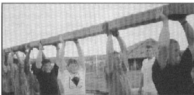
Soldiers work together to build a hospital in Kampong Cham.
