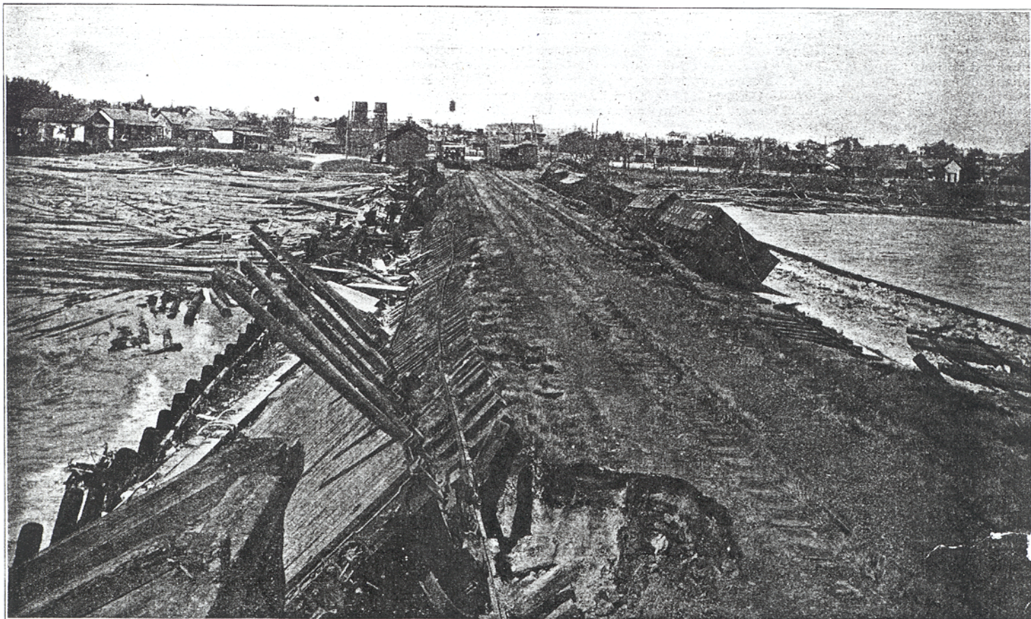
FIG. 3.—The effect of the storm at Pensacola, Fla.; view northward from Muscogee wharf, showing the effect of the high seas on the embankment.
