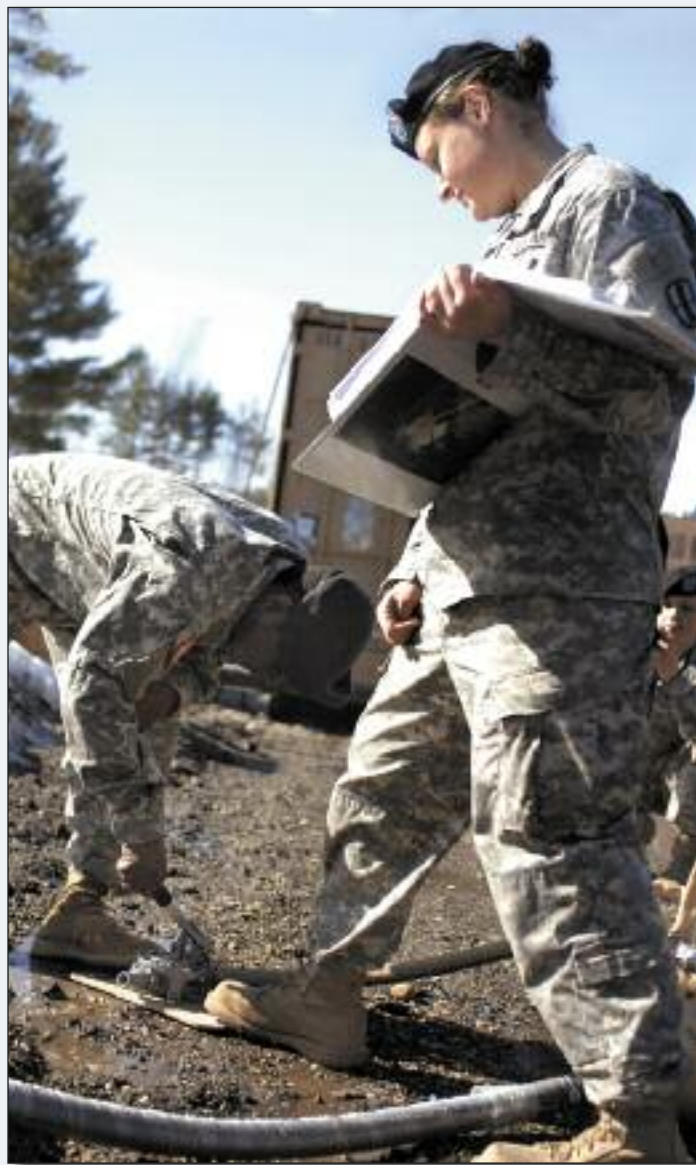
Pfc. Willie Barron and Pvt. Sara McPherson, of A Company, 3643rd BSB, set up the NHARNG's new water purification equipment at the water treatment plant in Somersworth, March 15. Photo: Staff Sgt. Ginger Dempsey, NHNG-PA
