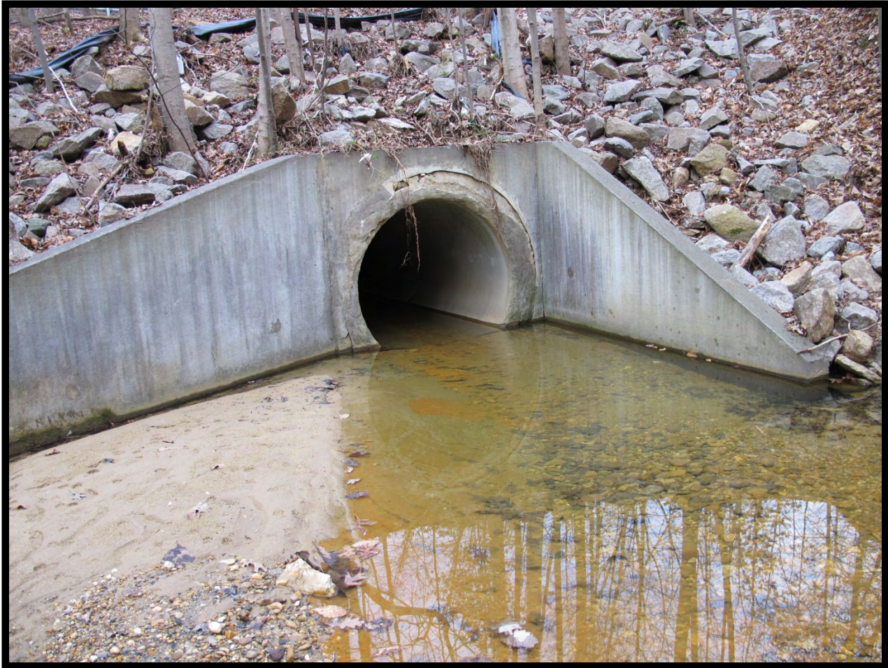
Figure 4.2-24: View of Culvert Under Route 1 (VDHR # 029-5712), Facing Northeast.
