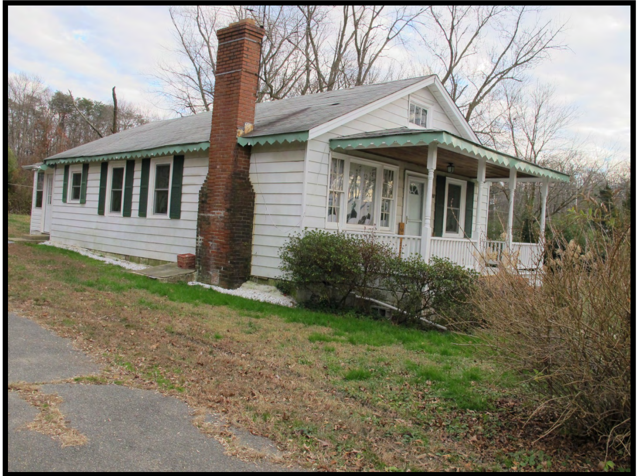
Figure 3.2-25: View of 9123 Shepherd Lane (VDHR # 029-5704), Facing Southeast.
