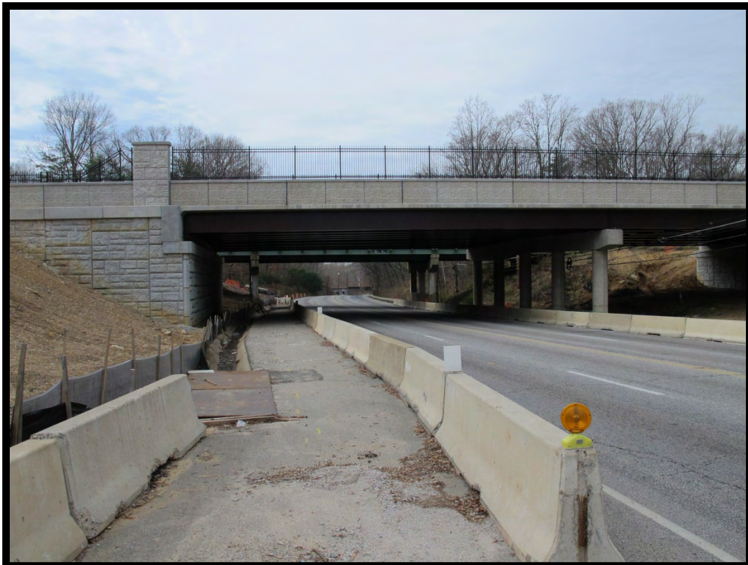
Figure 4.2-17: View of Route 1, (Old) River Road (VDHR # 029-5708), Towards Vehicle Bridge (Facility No. 1443, VDHR # 029-5425), Facing West. Note Vehicle Bridge is (VDHR # 029-5425) the Bridge in the Background.
