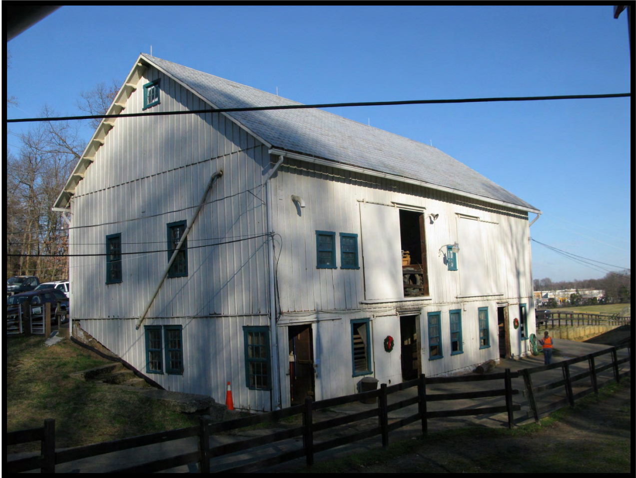
Figure 4.2-3: View of Bank Barn at the Sharpe Stable Complex (VDHR # 029-5181-0005), Facing Northeast.
