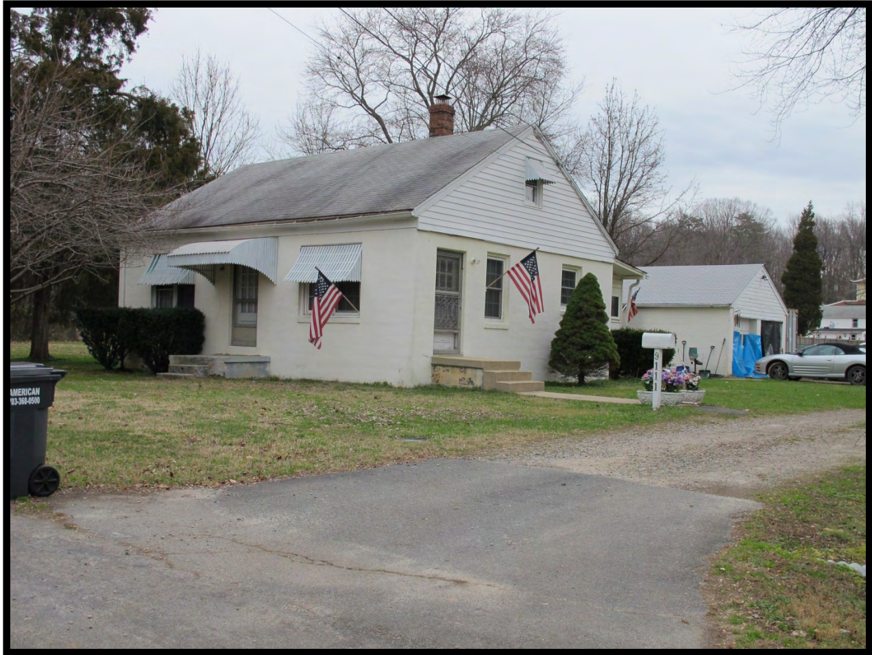
Figure 3.2-5: View of 9111 Anderson Lane (VDHR # 029-5685), Facing Northeast.
