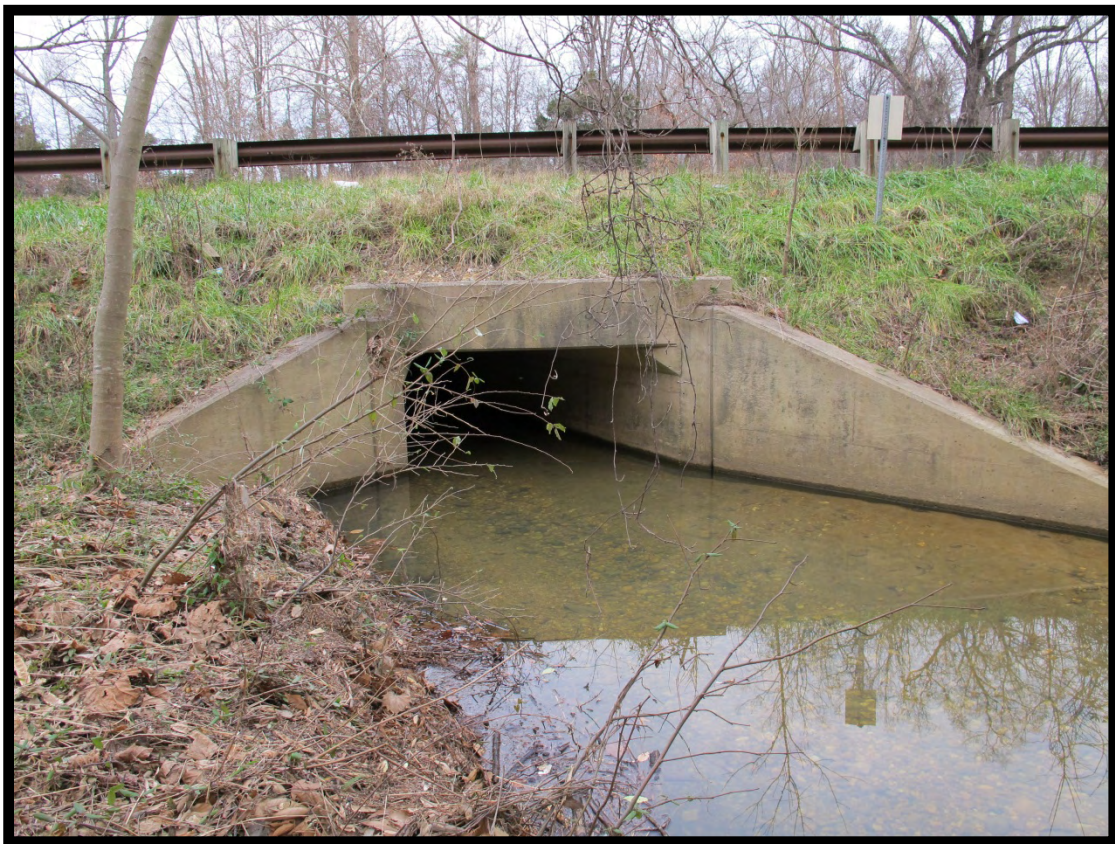
Figure 4.2-23: View of Culvert Under Route 1 (VDHR # 029-5711), Facing North.
