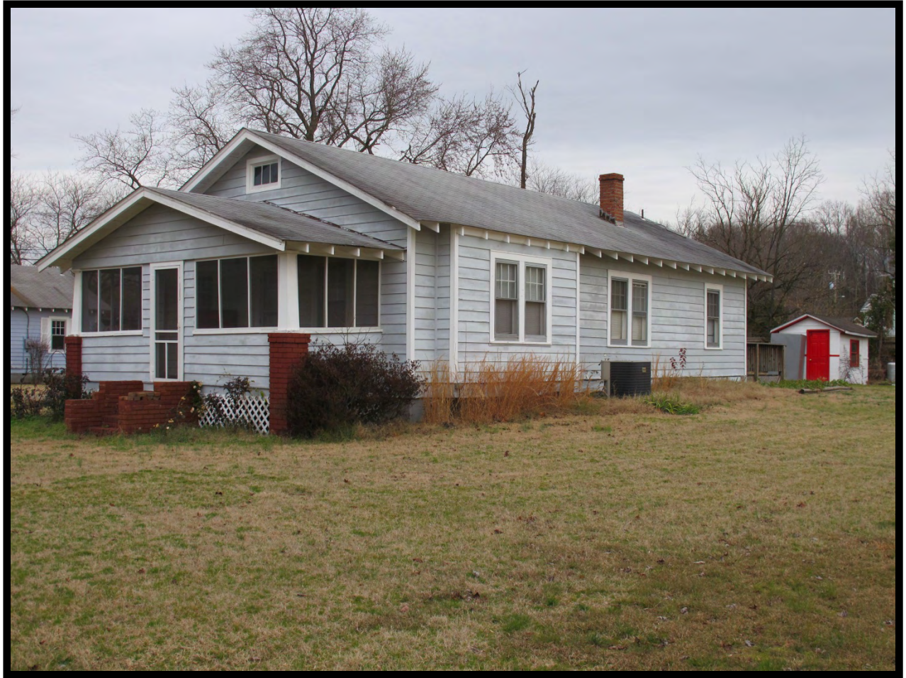
Figure 3.2-8: View of 9119 Anderson Lane (VDHR # 029-5688), Facing Northeast.
