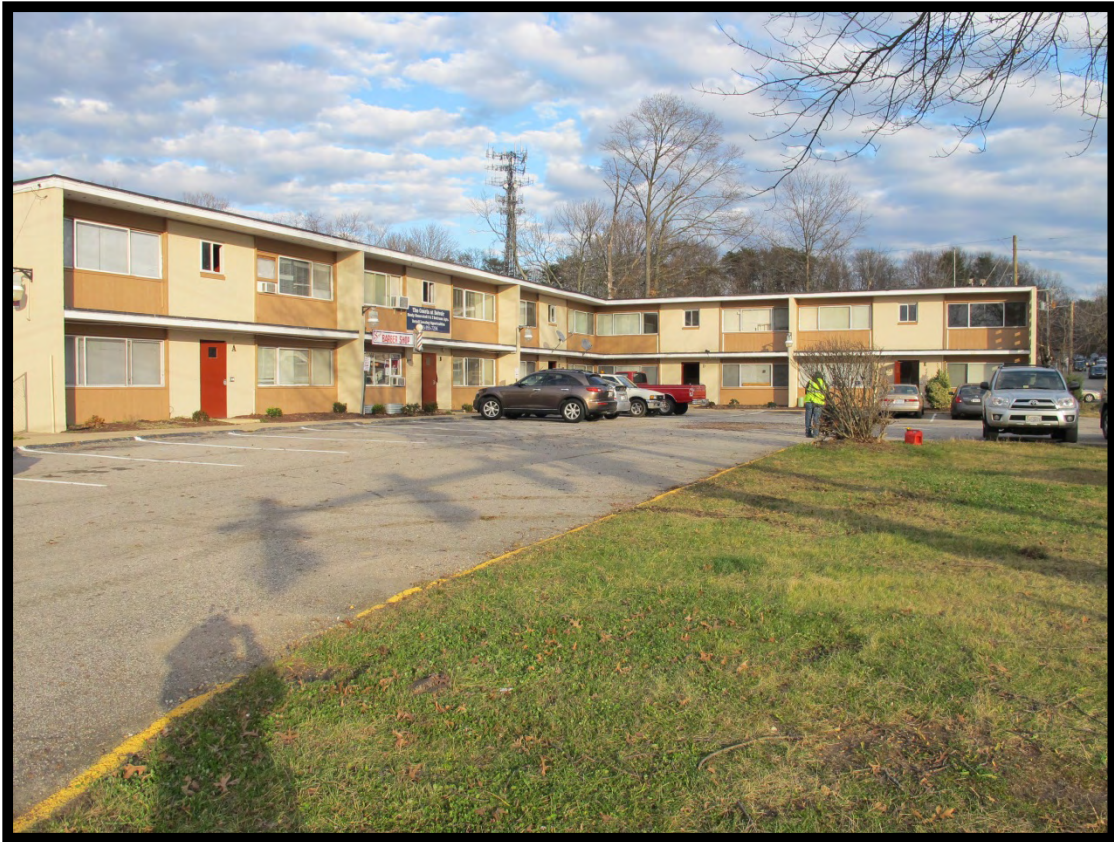
Figure 3.2-1: View of The Courts at Belvoir (VDHR # 029-5682 – South Block), Facing Northeast.
