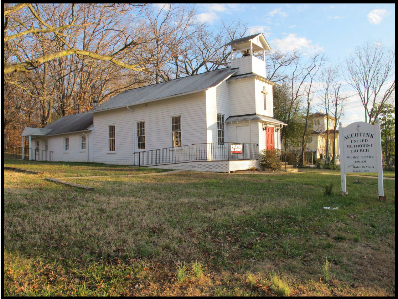
Figure 3.2-17: View of Accotink Methodist Church (VDHR # 029-5697), 9043 Backlick Road, Facing Southeast.
