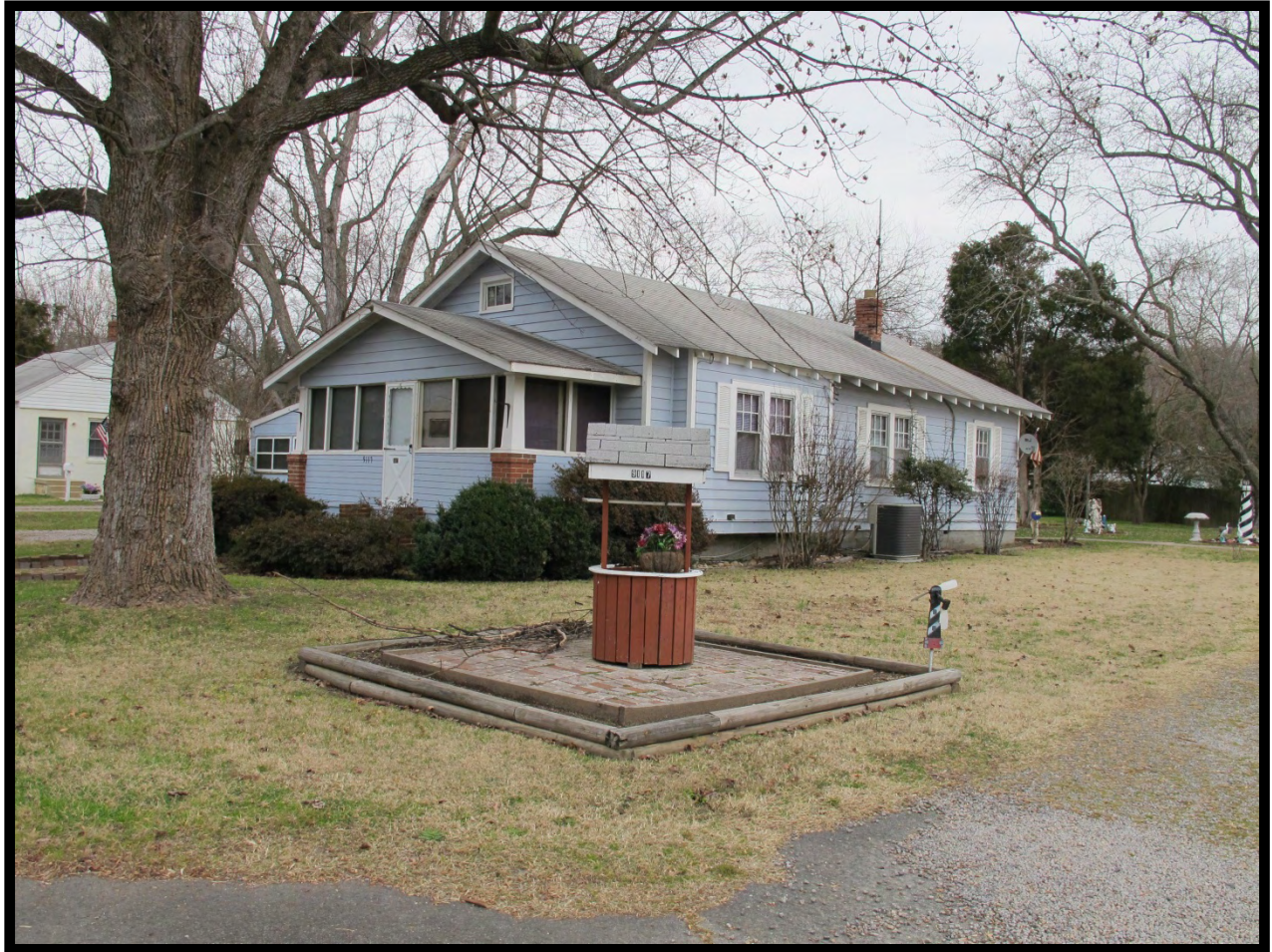
Figure 3.2-7: View of 9117 Anderson Lane (VDHR # 029-5687), Facing Northeast.
