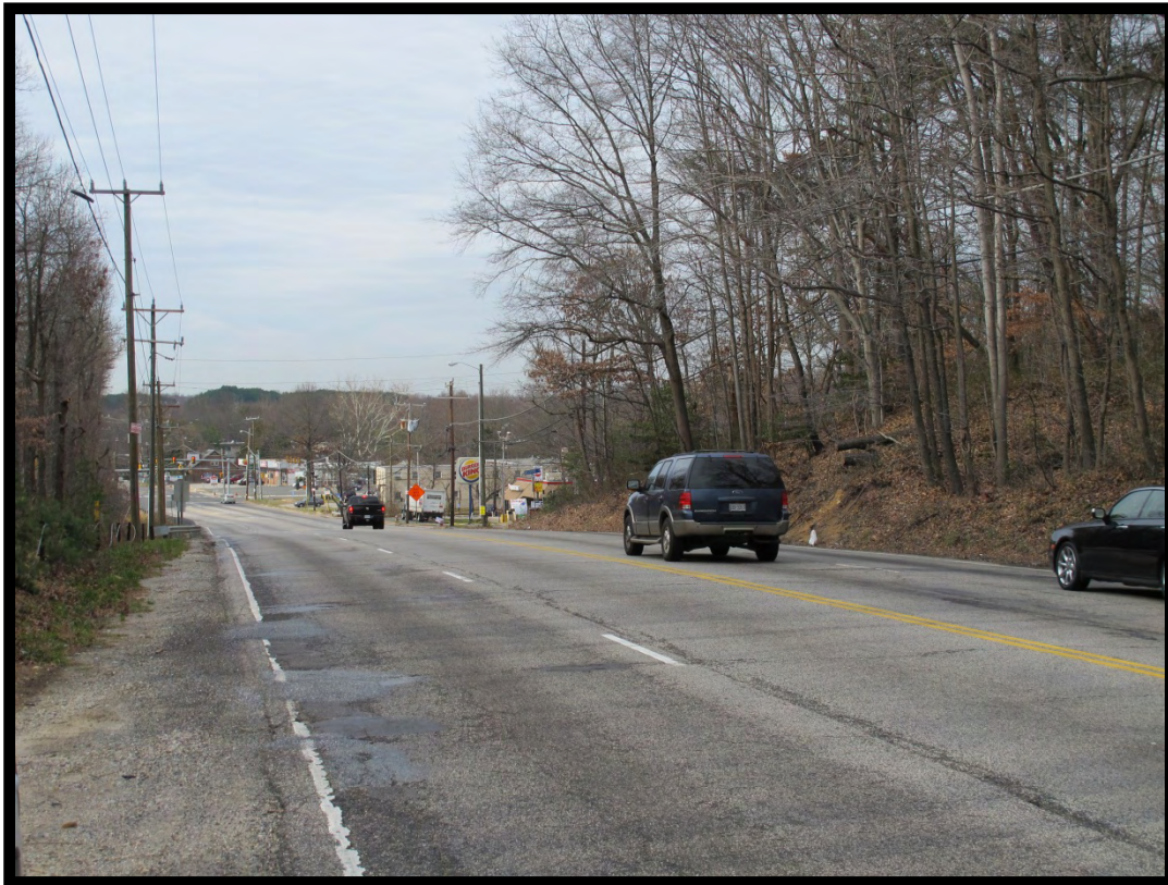
Figure 4.2-16: View of Route 1, (Old) River Road (VDHR # 029-5708), Towards Accotink, Facing West.
