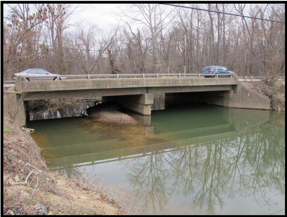
Figure 4.2-21: View of Bridge over Accotink Creek (VDHR # 029-5709), Facing Northeast.
