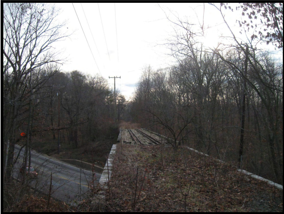
Figure 2.4-3: View of the Fort Belvoir Military Railroad Track Bed at Route 1 Crossing (VDHR # 029-5648), Facing Southeast.
