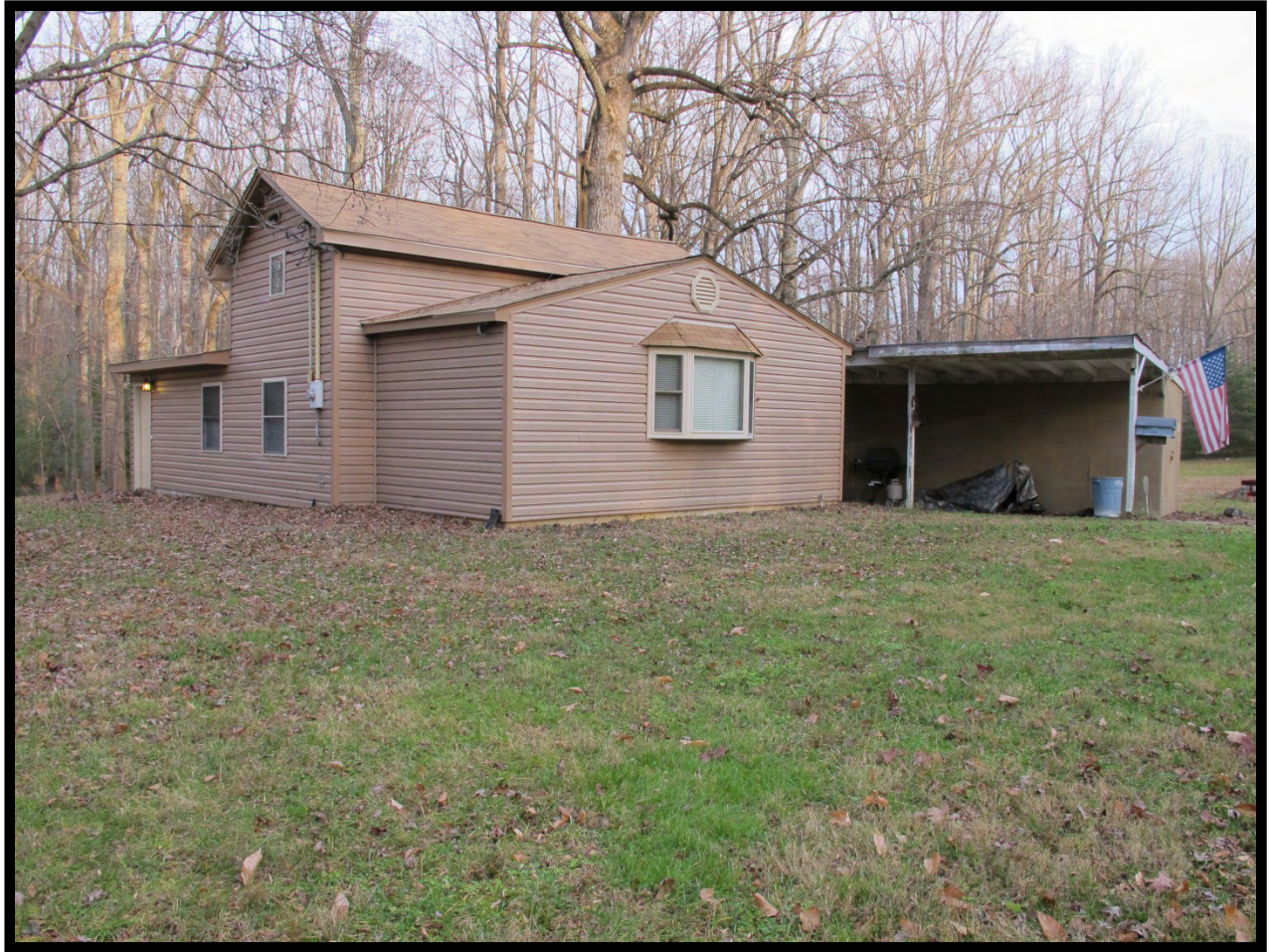
Figure 4.2-10: View of 9300 Old Colchester Road (VDHR # 029-5681), Facing Northwest.
