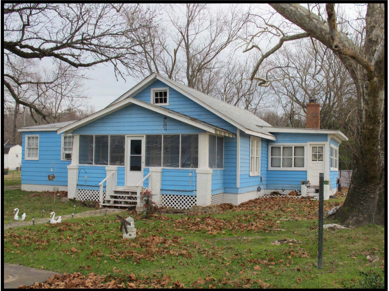
Figure 3.2-10: View of 9135 Anderson Lane (VDHR # 029-5690), Facing Northeast.
