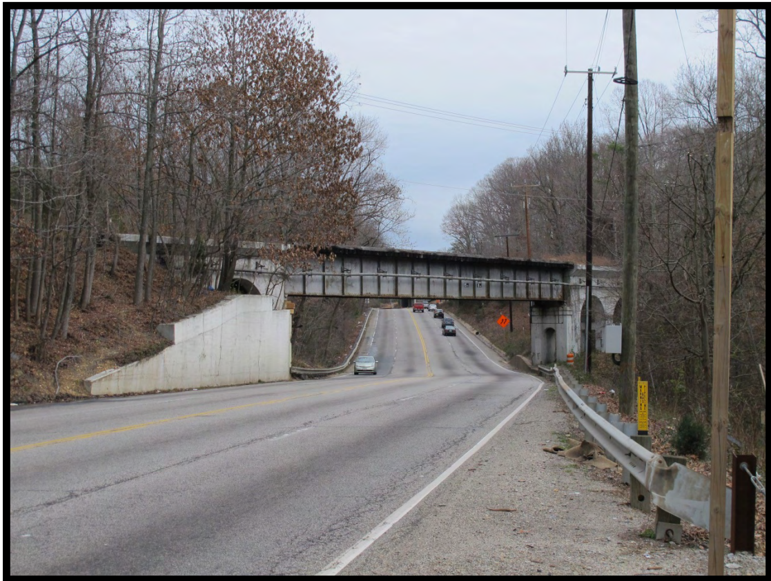
Figure 4.2-15: View of Route 1, (Old) River Road (VDHR # 029-5708), Towards Railroad Bridge (Facility No. 1433, VDHR # 029-5424), Facing East.
