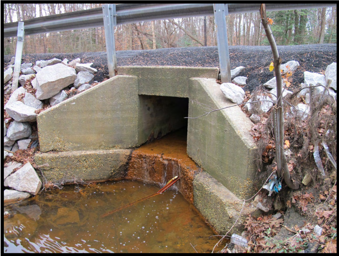
Figure 4.2-22: View of Culvert Under Route 1 (VDHR # 029-5710), Facing Northwest.
