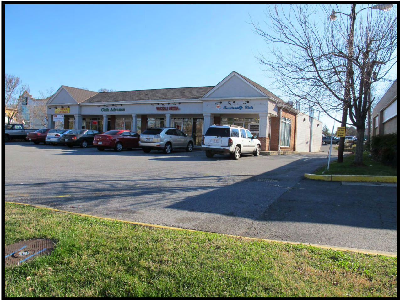
Figure 4.2-11: View of 8853-59 Richmond Highway (VDHR # 029-5705), Facing Southeast.
