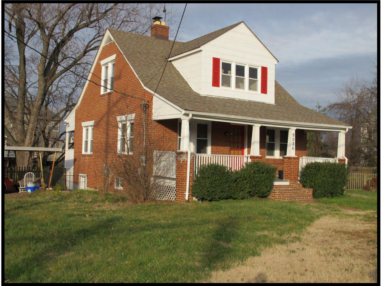
Figure 4.2-9: View of 9036 Telegraph Road (VDHR # 029-5680), Facing Northwest.
