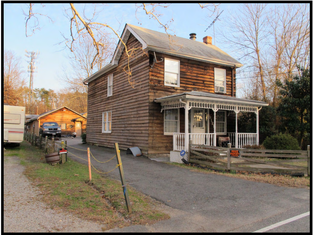
Figure 3.2-23: View of 9121 Backlick Road (VDHR # 029-5702), Facing Southeast.
