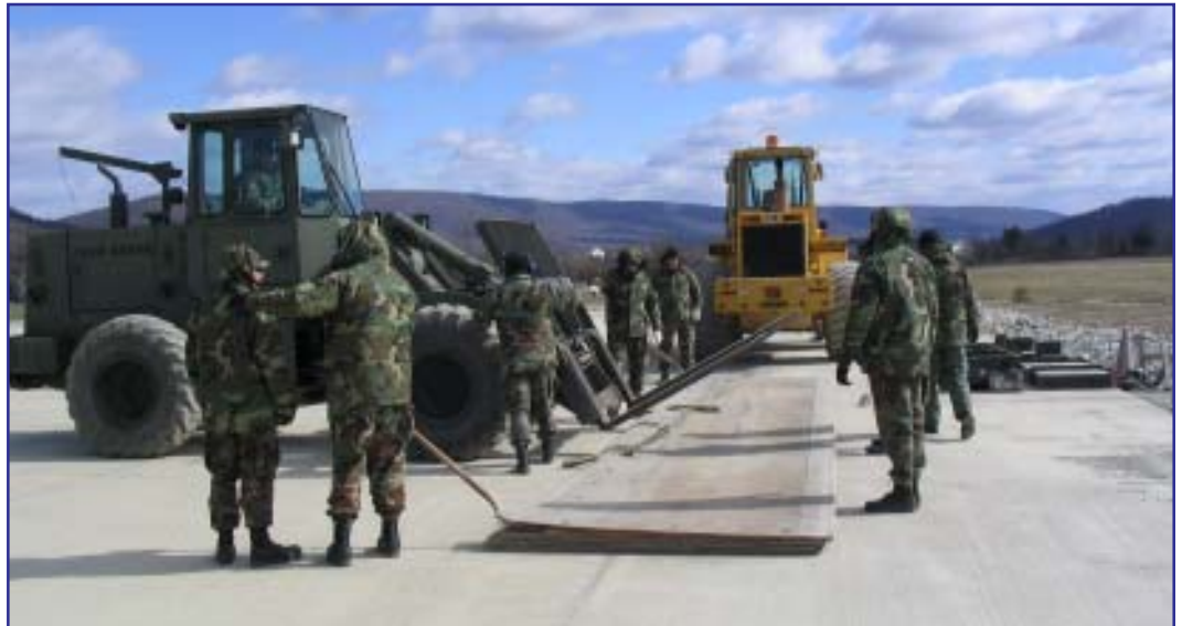
Tech. Sgt. Kenneth Bowman, Tech. Sgt. Thomas Jones, Master Sgt. Brian Kirby, Master Sgt. John Cody, Senior Airman Christian Zuniga, and Master Sgt. Joseph Collins assemble fiberglass matting as part of rapid runway repair operations.
