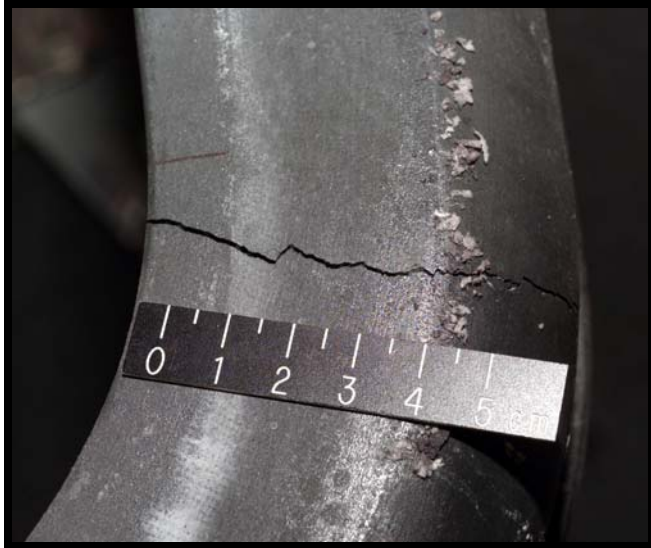
Figure 2. Through crack on lock-side rib of RCC panel 6. The crack propagated across the entire rib, the lock, and onto the lower surface of the panel. The total crack length is 14 cm.
