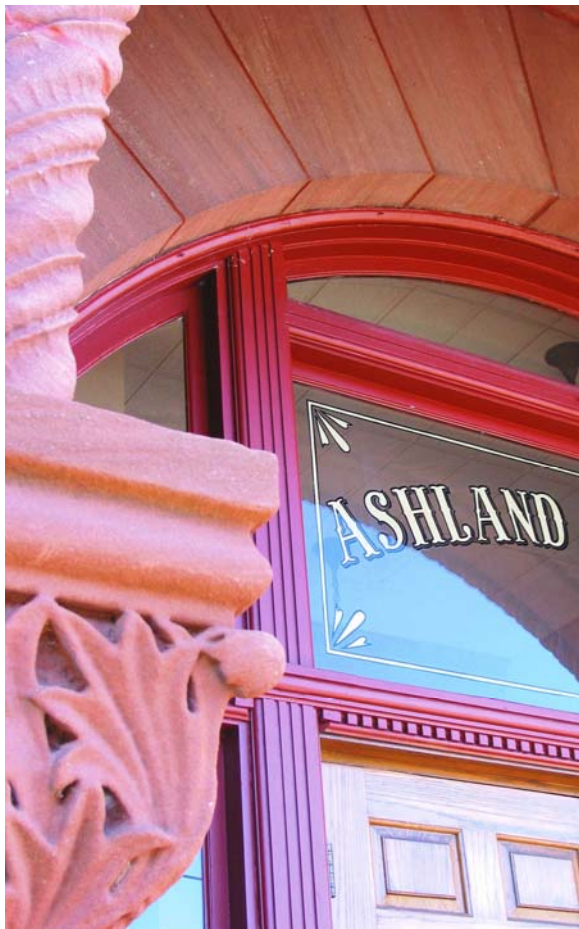
Ashland City Hall Source: City of Ashland
