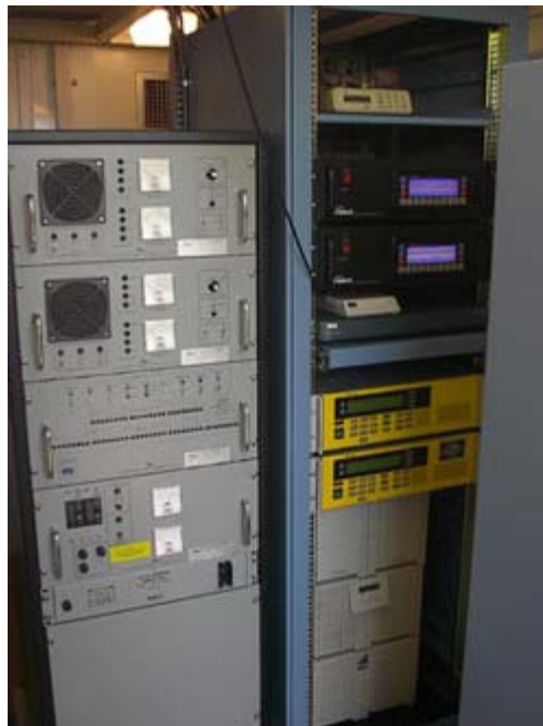
Figure 1. Hagerstown—The HA-NDGPS Broadcast Station Rack
