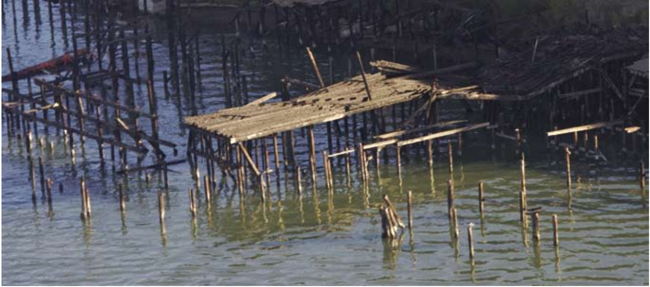
A derelict creosote piling structure slowly falls into the bay.
