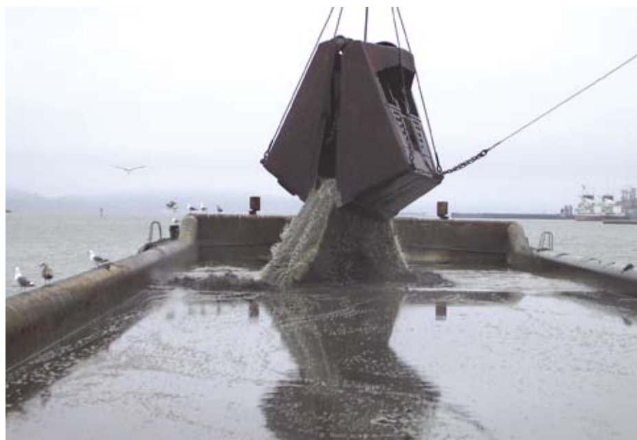
Maintenance dredging at the Port of Richmond.
