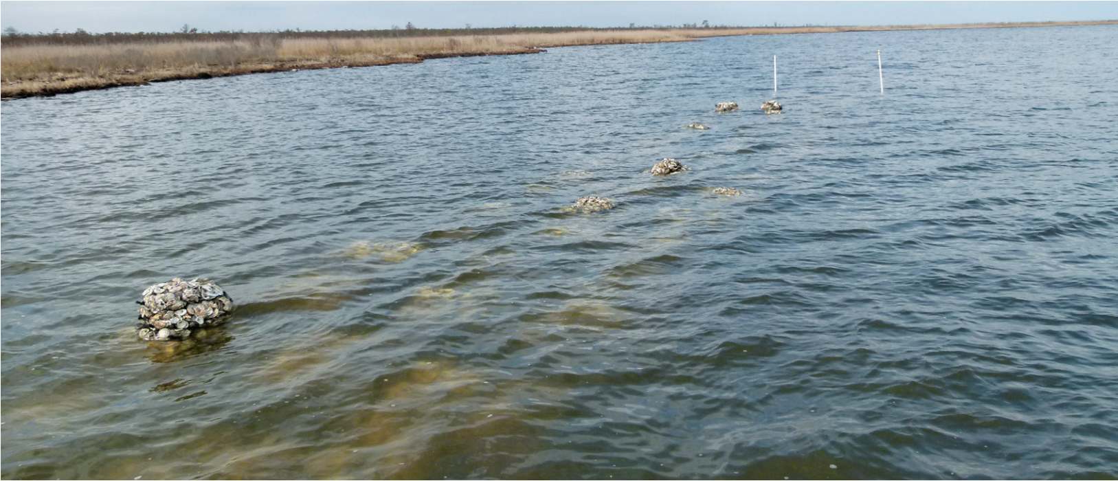
Shoreline protection reef after deployment of bagged oyster shells. © Aaron McCall, TNC
