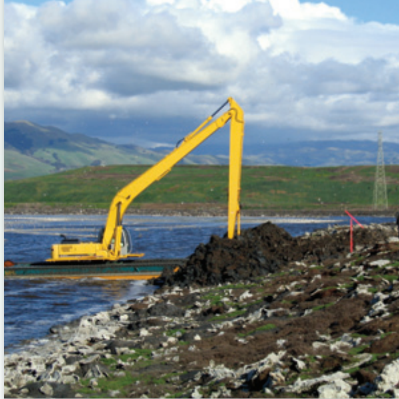
TOP LEFT: AFTER BAY WATER EVAPORATES, INHOSPITABLE, BARREN SALT FLATS ARE LEFT BEHIND. MIDDLE: AFTER RESTORATION, THOSE BARREN FLATS BECOME WETLANDS AGAIN. ABOVE RIGHT: A DREDGE BEGINS THE WORK OF RESTORING A SALT POND. All photos courtesy of the California Coastal Conservancy
