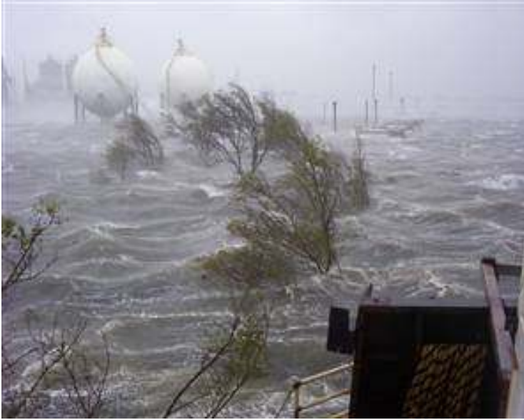
Figure 3: Storm Surge and Flooding Post-Katrina at Petrochemical Facility
