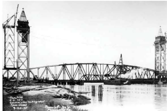
1935 construction of the Cape Cod Canal Railroad bridge located in Bourne, Mass.
