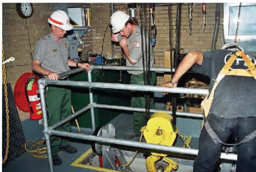
Park rangers perform repair work at Tully Lake, Royalston, Mass.
