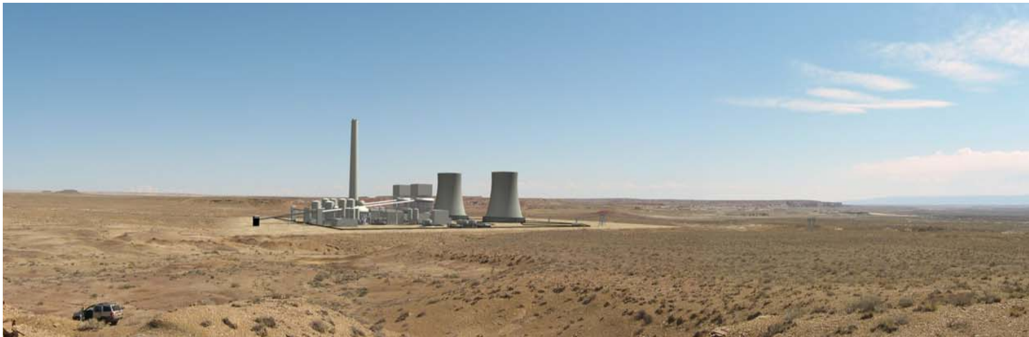
The power plant would dominate views from this location. Views of the horizon from this direction are blocked by the proposed power plant as simulated in the picture. This simulation represents the highest level of impact on sensitive viewers.
