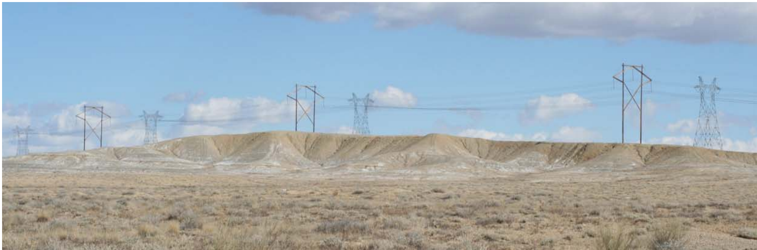
This simulation represents a view toward the existing transmission line facilities showing the proposed project. The tower type and construction materials help to make the proposed structures less dominant than the existing transmission line. However, the backdropping of the project against the sky still renders it more visible resulting in moderate to moderate-high impacts from this viewpoint.
