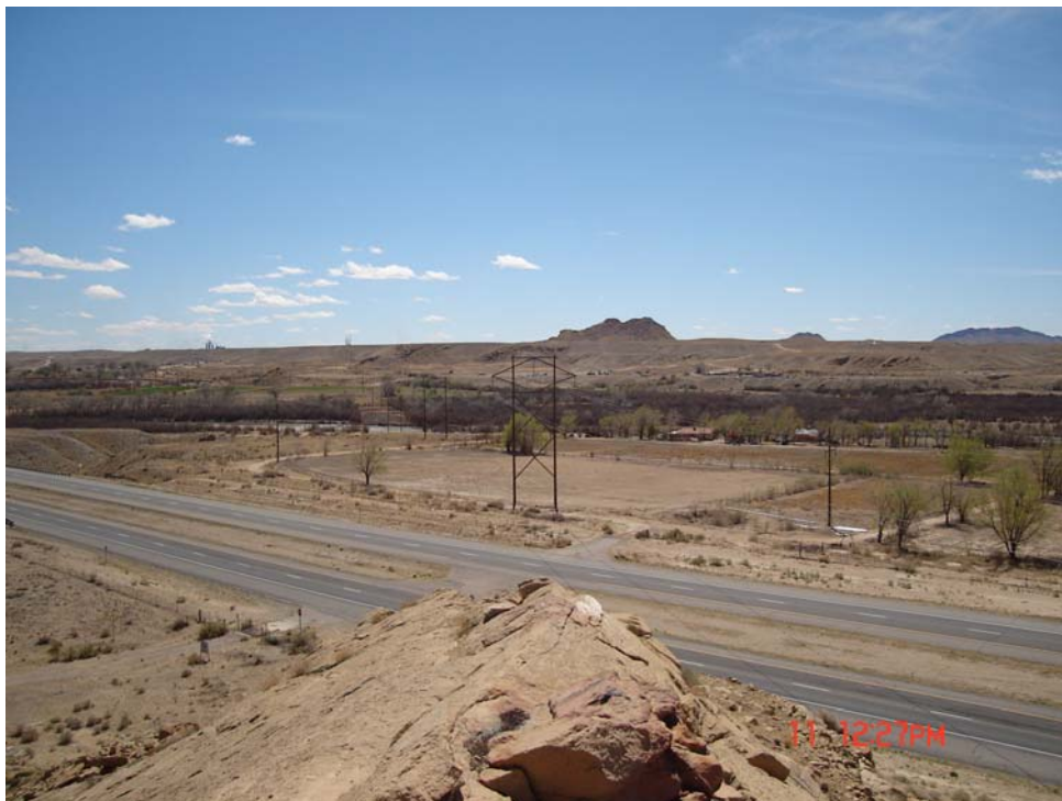
Figure 2. Transmission Line proposed San Juan River crossing, looking south across U.S. Highway 64 onto the floodplain.
