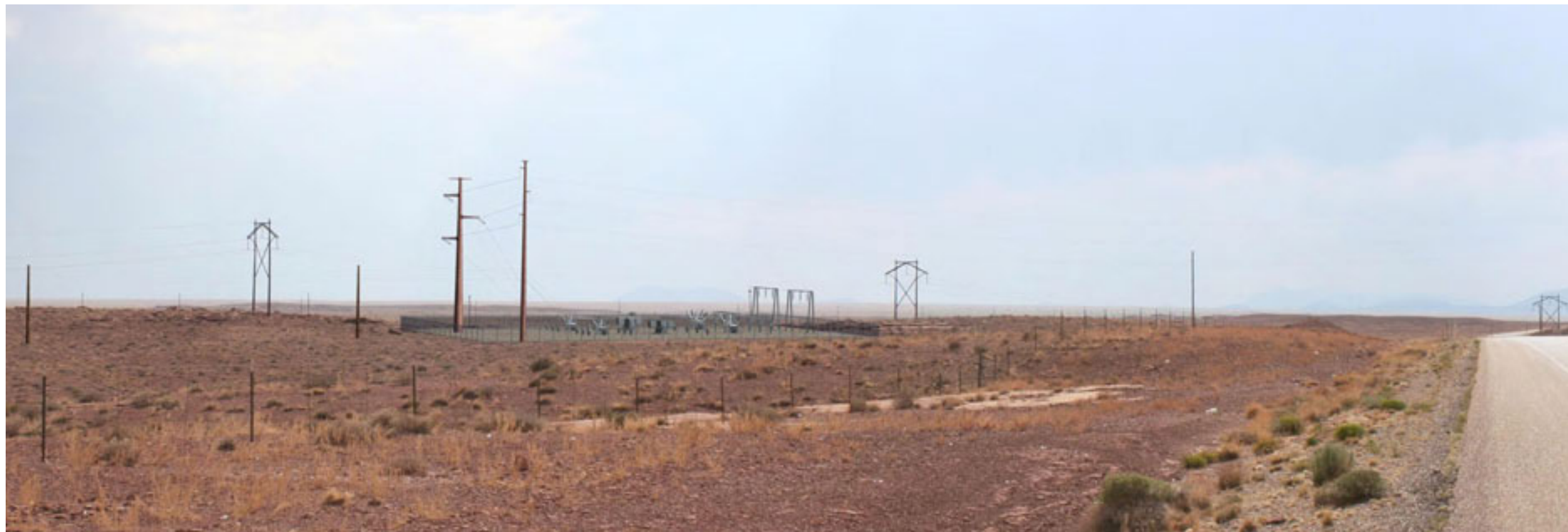
Simulation: Proposed substation with accompanying 69kV Corten single pole structures and 24.5kV wood pole structures
