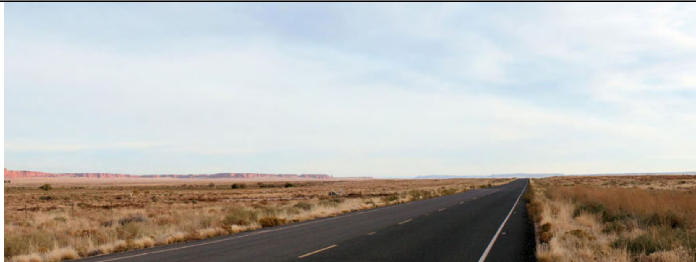
Existing Conditions: View northeast along Indian Route 2 at Milepost 30 of the water-supply pipeline route
