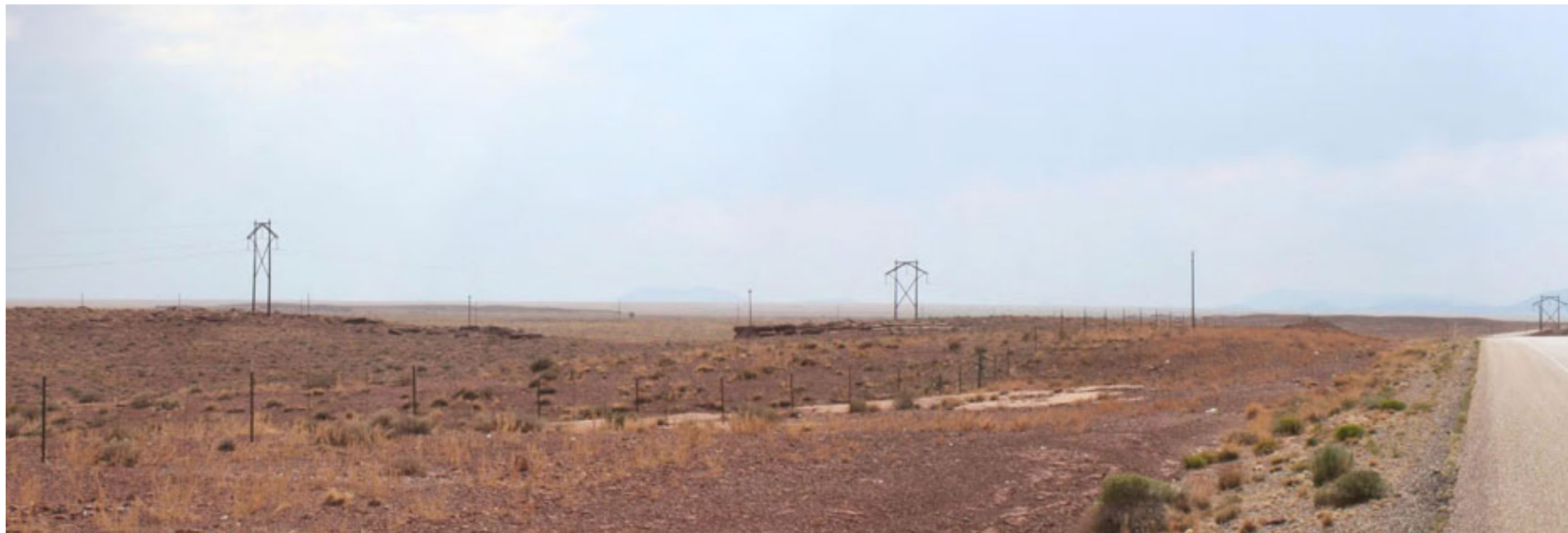
Existing Conditions: View west on State Route 99 at location of existing 230kV transmission line
