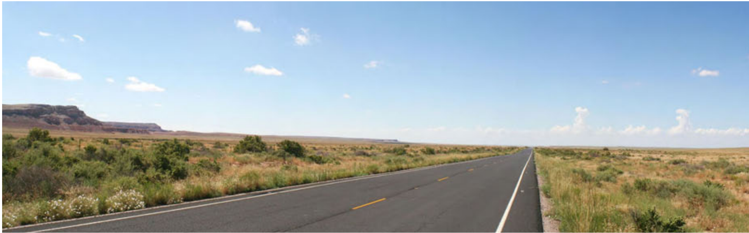
Existing Conditions: View southwest along Indian Route 2 at milepost 45.5 of the water-supply pipeline route
