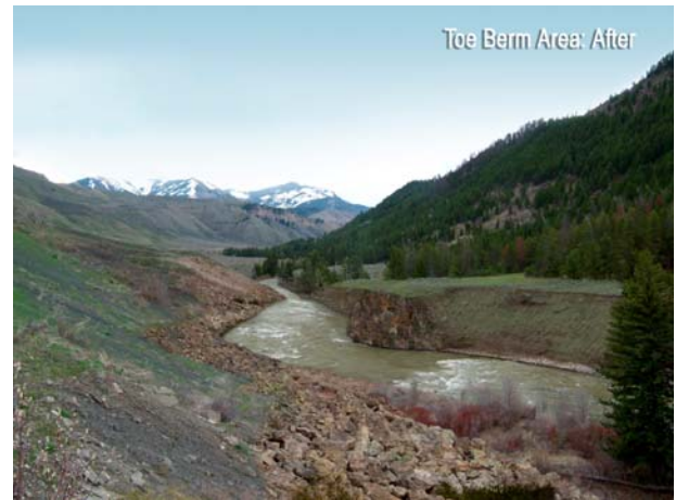
Figure 5: Toe Berm Area - After
