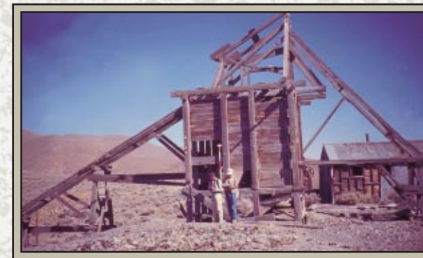
A Vertical Shaft. Such shafts may open directly to vertical drops of several hundred feet.
