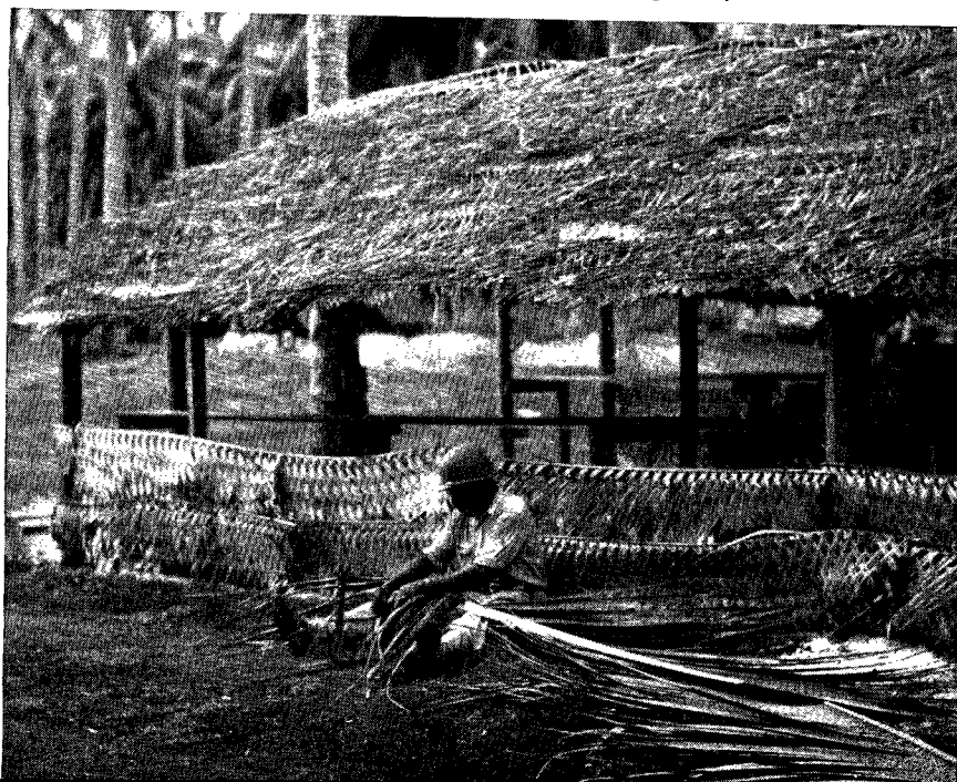
A butcher knife snatched from the mess hall helps this colored soldier expertly weave the walls of a new building from palm fronds.
