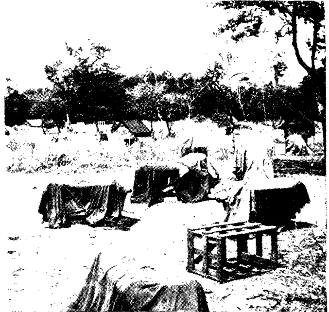
An excellent job of garnishing is being done on this drape job over an operations tent of a heavy bombardment group. The net has been spread so that outlines are vague when seen from the air and the garnish has been dyed to blend well with the terrain. No telltale shadows are cast.
