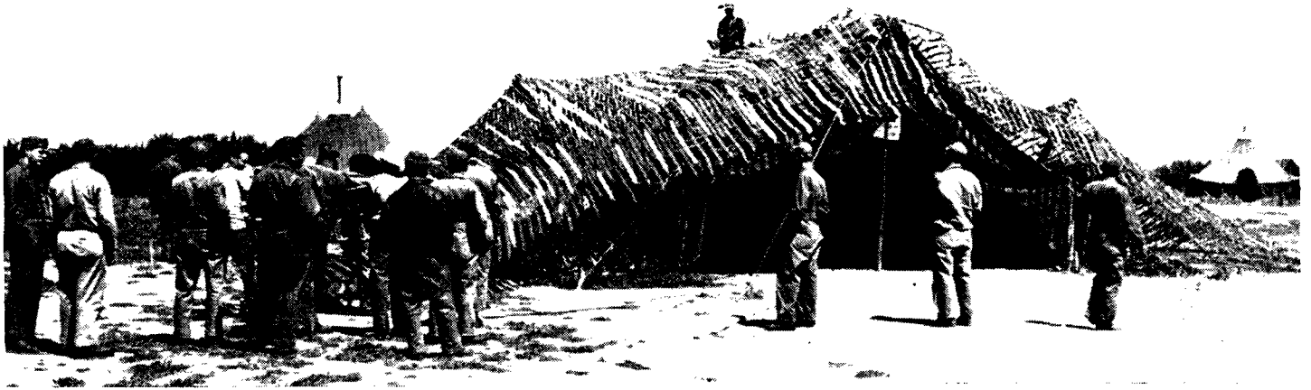
An excellent job of garnishing is being done on this drape job over an operations tent of a heavy bombardment group. The net has been spread so that outlines are vague when seen from the air and the garnish has been dyed to blend well with the terrain. No telltale shadows are cast.
