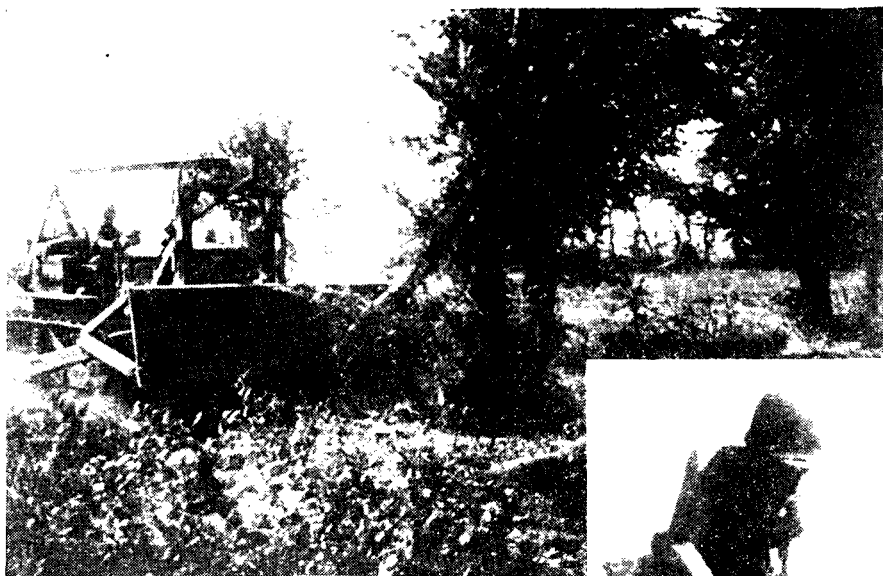
Establishment of airfields was of first importance. Just one mile from the beach aviation engineers selected two adjoining farms for conversion into an emergency landing field. Trees were bulldozed and a fast job with pick axes helped level off the new runway. First to use the field were two P-38s which came in exactly 24 hours after the cotton and wheat fields were taken over by aviation engineers. The task of engineers in advancing our airbases closer to the enemy and his supplies is vital in maintaining control of the battle sky.
