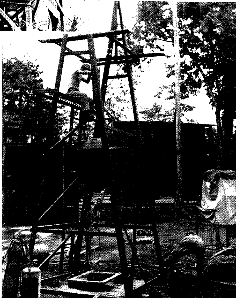
The newest addition to the Gunnery School is the belly turret which is being hoisted to the top of a tall scaffold which was designed to provide the belly gunner with the firing angle he will ordinarily encounter in actual aerial combat.
