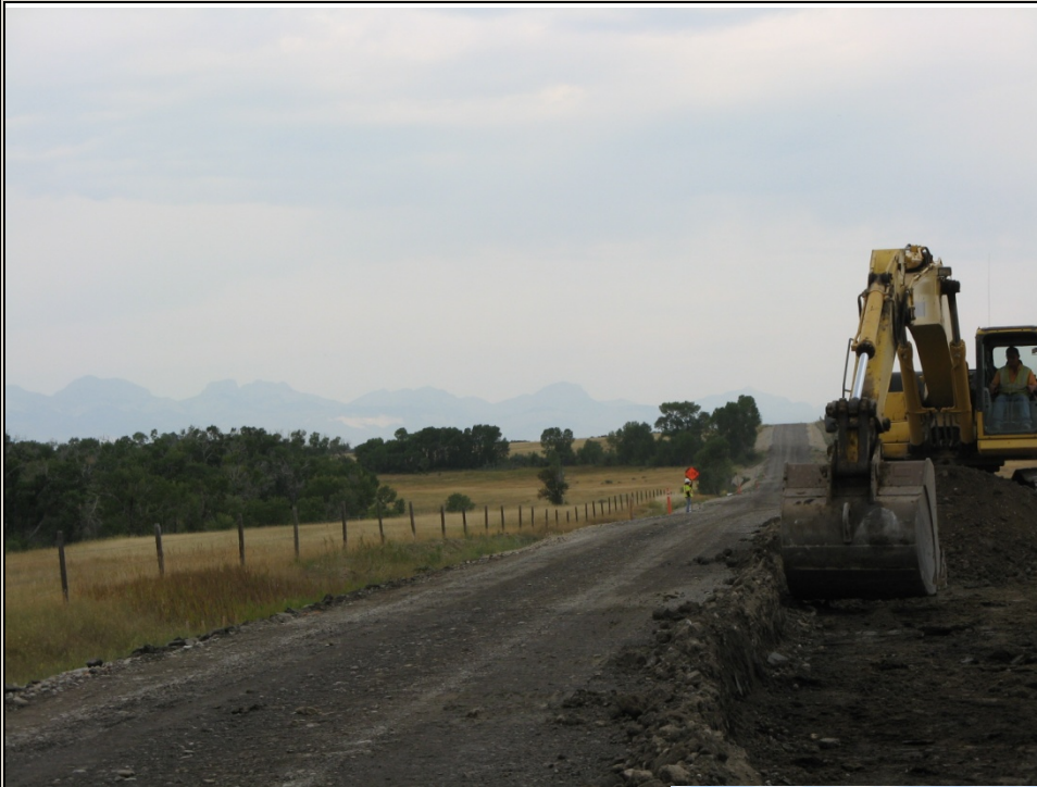
Subexcavation of unsuitable material nears Spring Hill.
